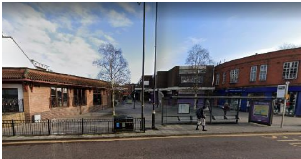
Figure 17: Looking east into the original entrance of the Longfield Centre from Bury New Road, showing the c1930s shops to the right, 1960s precinct buildings to the centre and c1990s building to the left. This view illustrates the poor pedestrian environment experienced at this principal entrance point.
