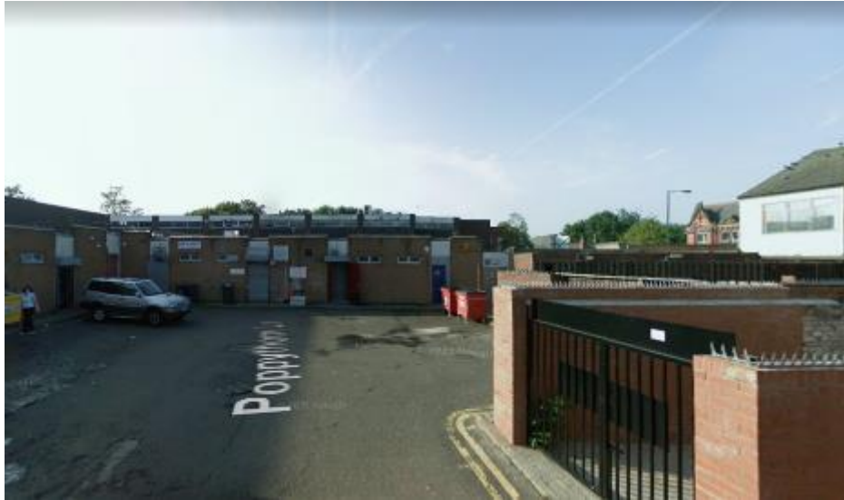
Figure 18: A view looking into the service yard of the 1960s shops that form part of the original Longfield Centre, illustrating the poor back of house spaces that are fully visible from the principal public realm to the north (behind).
