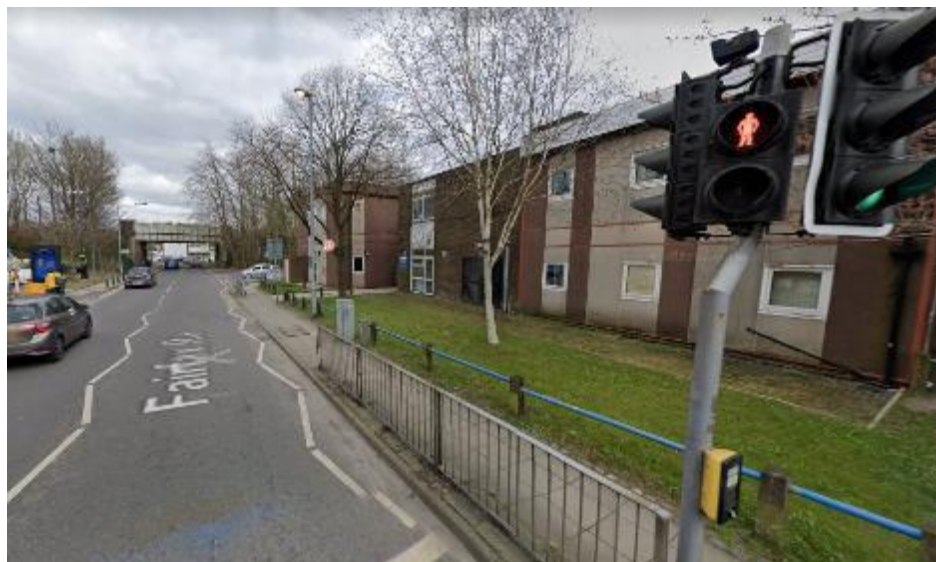
Figure 23: A view looking north-east along the northern end of Fairfax Road towards the railway line and bridge to the distant left. This view illustrates the low quality c1970s Prestwich Health Centre, which is located on the north-western corner of the Site.
