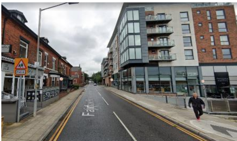
Figure 21: Looking north-east along Fairfax Road showing the Radius apartments to the right, and a row of late-19 th century terraced housing to the left. To the distant left can be seen the locally listed Our Lady of Grace Church, Hall and Presbytery.
