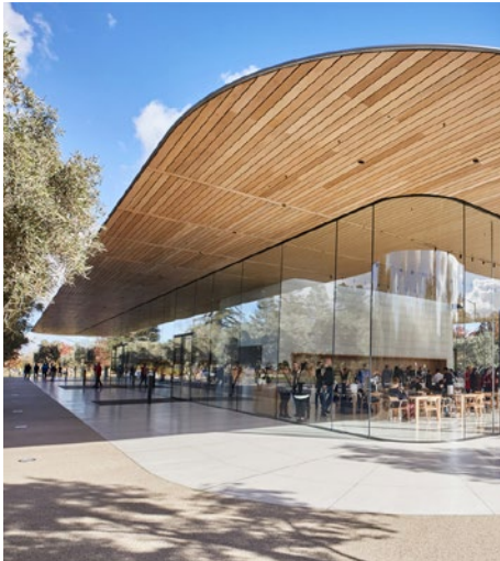
Feature timber soffit
