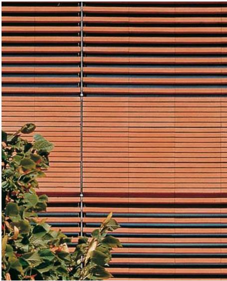
Ventilated terracotta cladding
