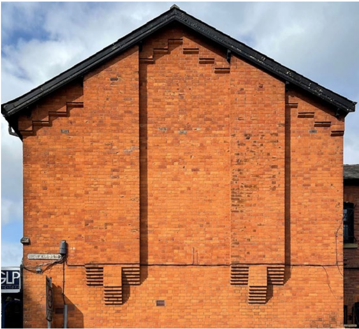
Gable, 9 Fairfax Road
