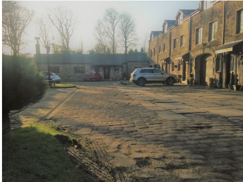
The Byre seen across the service courtyard
