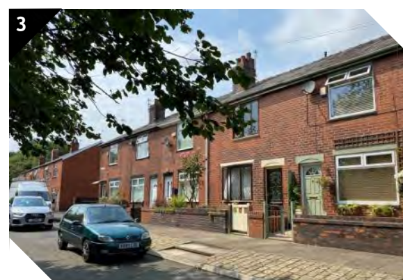
Terraced housing on Brook Street
