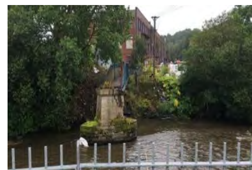
Figure 3.5: Photo of former bridge location
