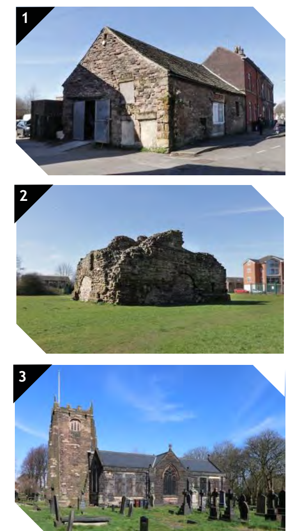
Figure 2.8: Photographs of Listed Buildings
