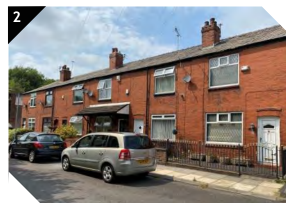
Terraced housing on Brook Street
