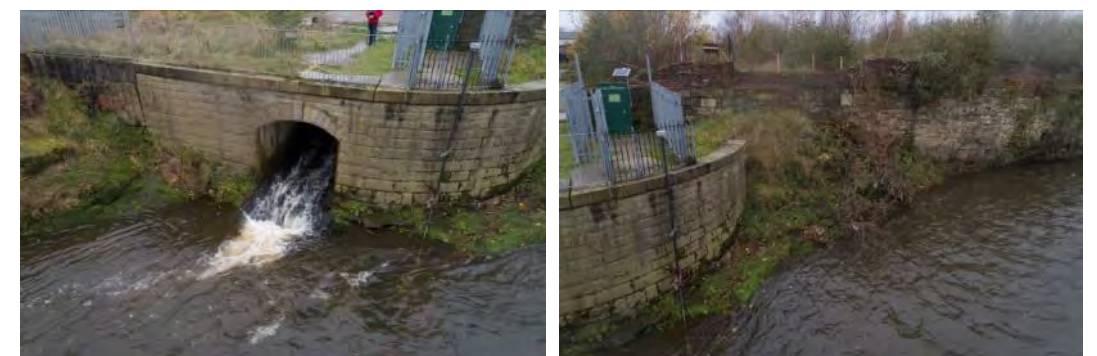
Figure 2.5: Photographs of existing river wall and the crow trees from brook culvert
