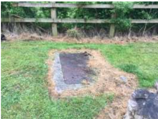
Plate 6: Sealed chambers located just outside the perimeter of the site. It is unknown what is contained inside.
