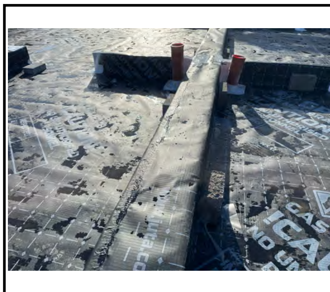
The JUTA GP1 Gas Barrier crosses the internal cavity to create a robust seal throughout.
