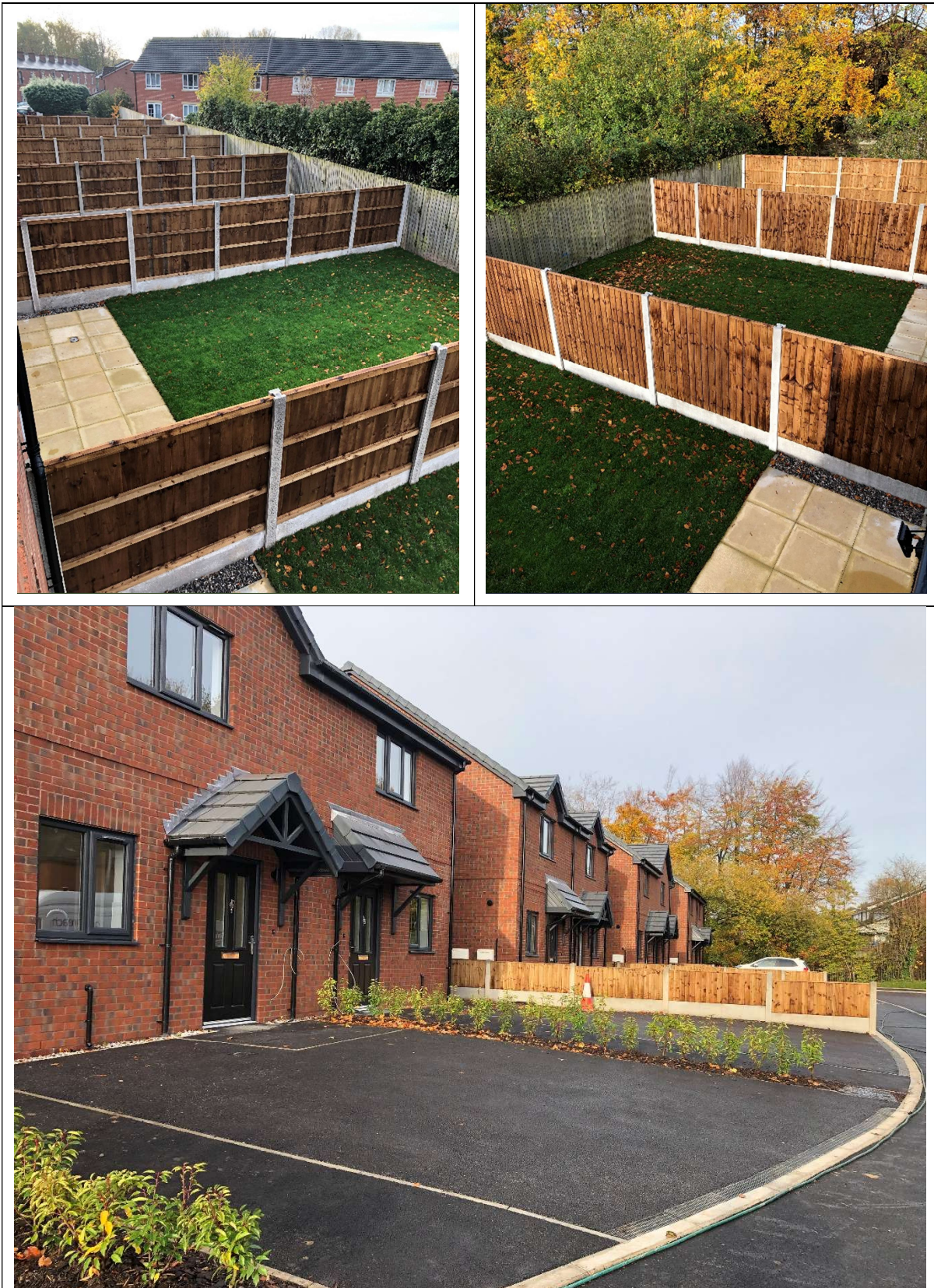
Photographs 1-3: Selected photographs of completed site.
