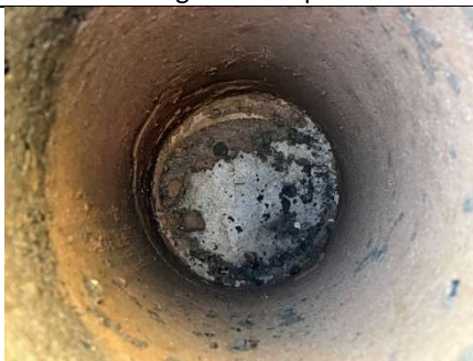
Downhole view of soil in capping layer excavation in rear garden area showing membrane.
