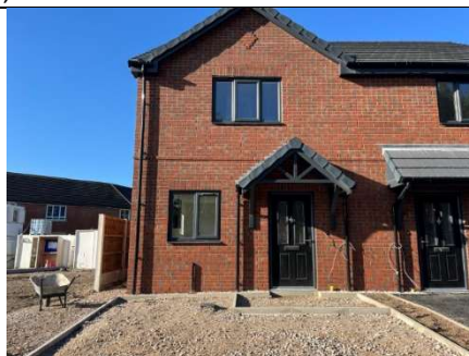
View of front showing small strip of soft landscaping.
