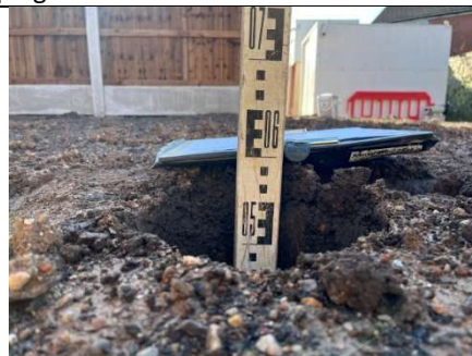
Depth measurement of the capping layer in rear garden (c.600mm).
