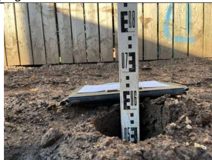
Depth measurement of the capping layer in rear garden (c.625mm).
