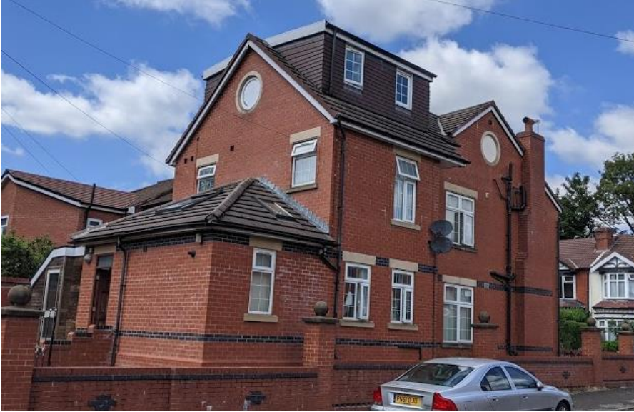
Prominent flat roofed box dormers at rear of 42 Richmond Avenue, corner plot property located on the corner of Richmond Avenue and Mildred Avenue.
