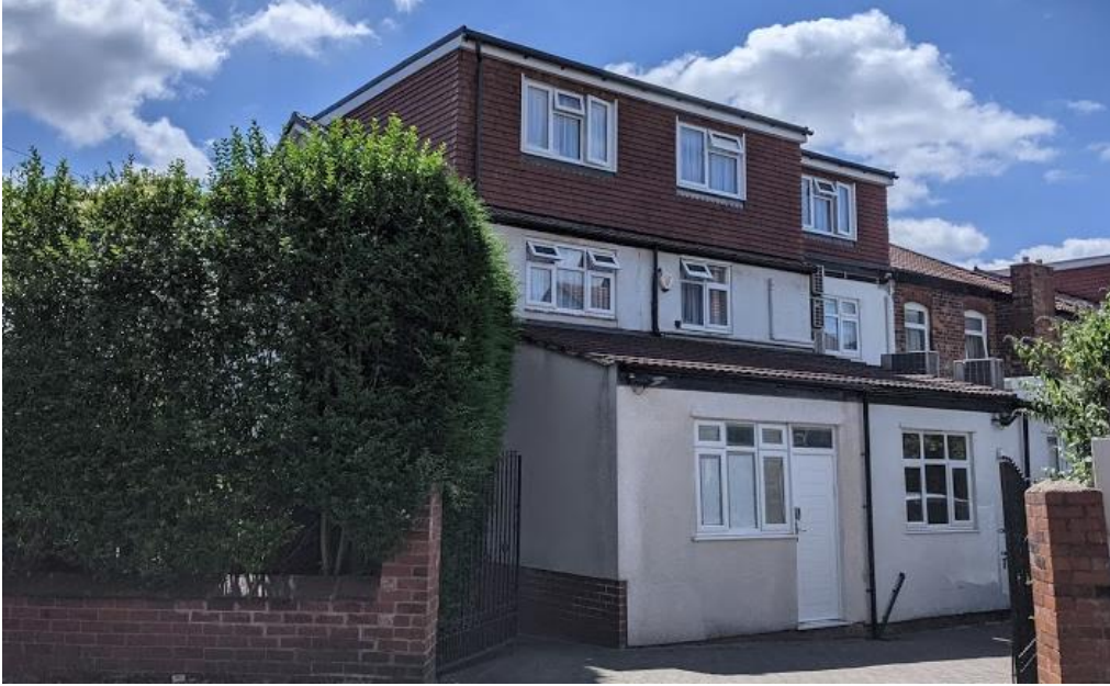
Prominent rear flat roofed box dormer at rear of 47 Kings Road, corner plot property located on the corner of Kings Road and Queens Drive.
