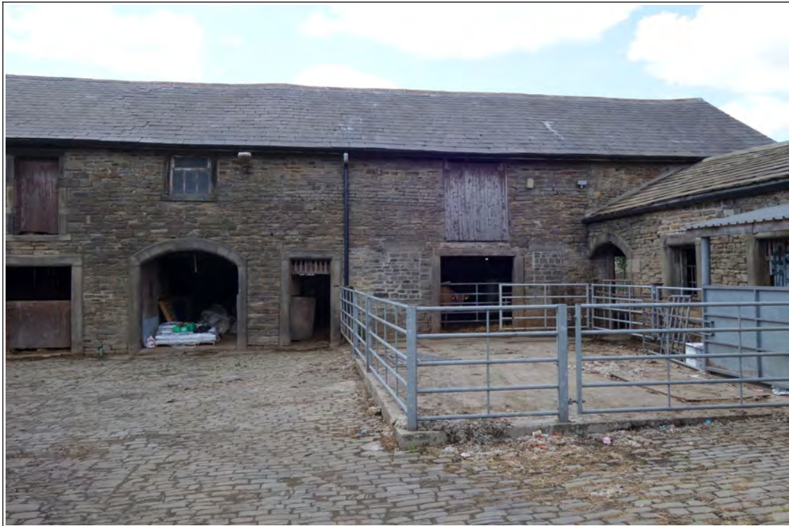
Photo 1: North-west corner of courtyard
