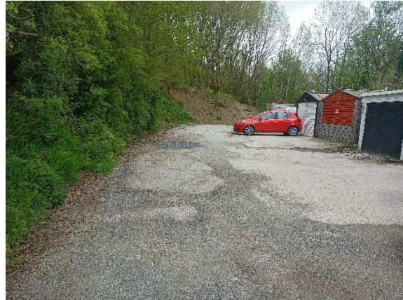
Photograph 2: Garage/parking area adjacent to the site.
