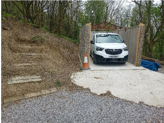
Photograph 1: Newly constructed garage building and adjacent bare ground ramp/path.
