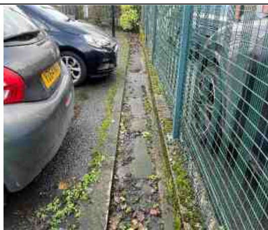
Photograph 8: Concrete drainage channel adjacent to George Street and S boundary.
