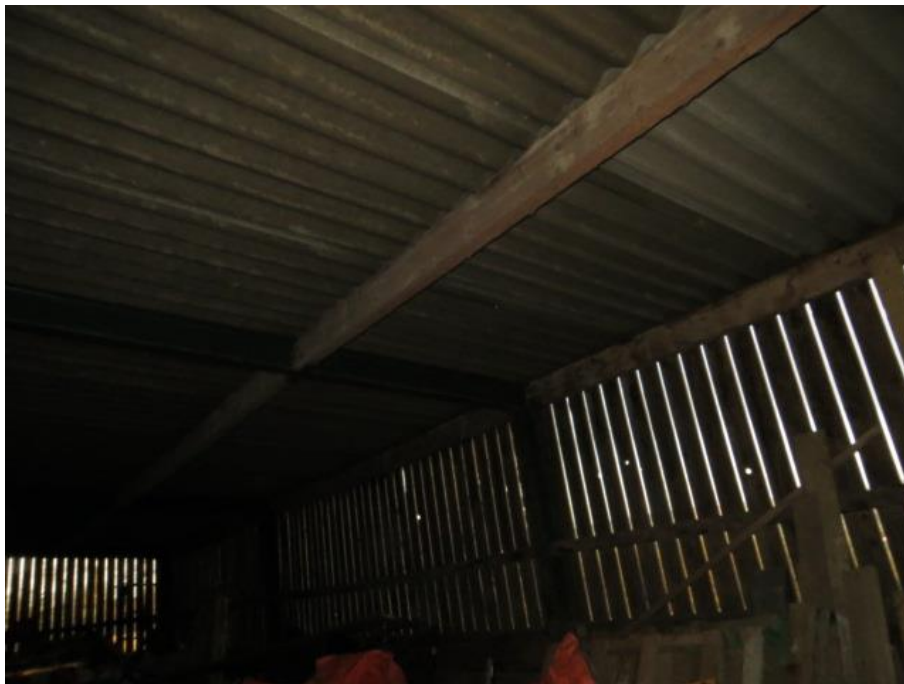
INTERNAL VIEW OF RIGHT HAND BARN
