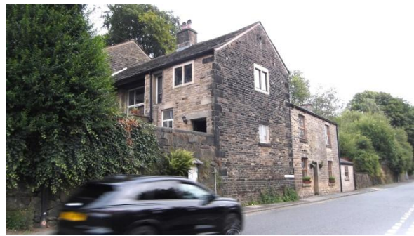
(14) Higher House Cottage/barn and 3 Helmsore Road
