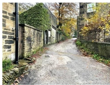
(22) Moor Road, watershot wall and gate
