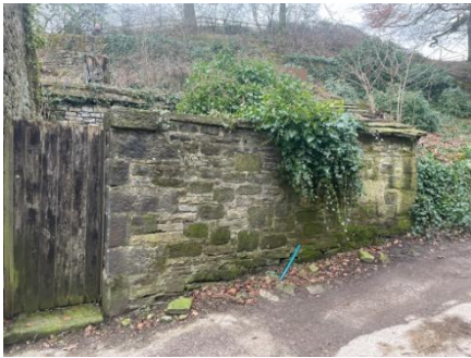
(21) Boundary wall in north
