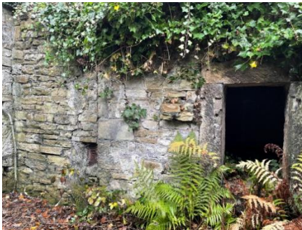
(24) Good quality tooled stone framing
