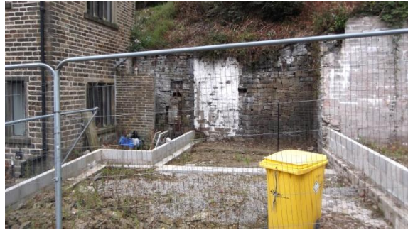
(16) Original stone retaining wall
