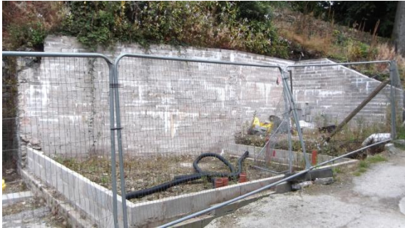
(17) New retaining and flanking wall
