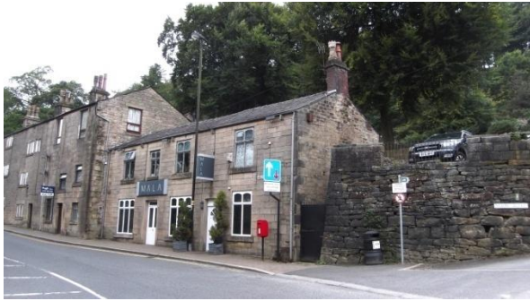
(13) 18 to 34 Holcombe Village
