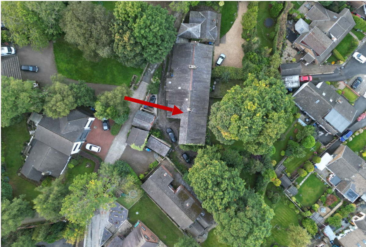
1.6b – 33 Sunny Bank Street – aerial photograph.
