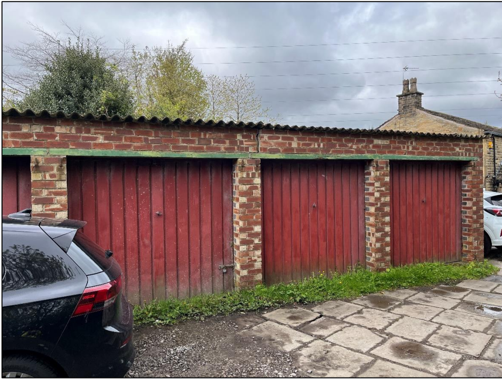
Plate 1 – Exterior of building B1 (brick garages)
