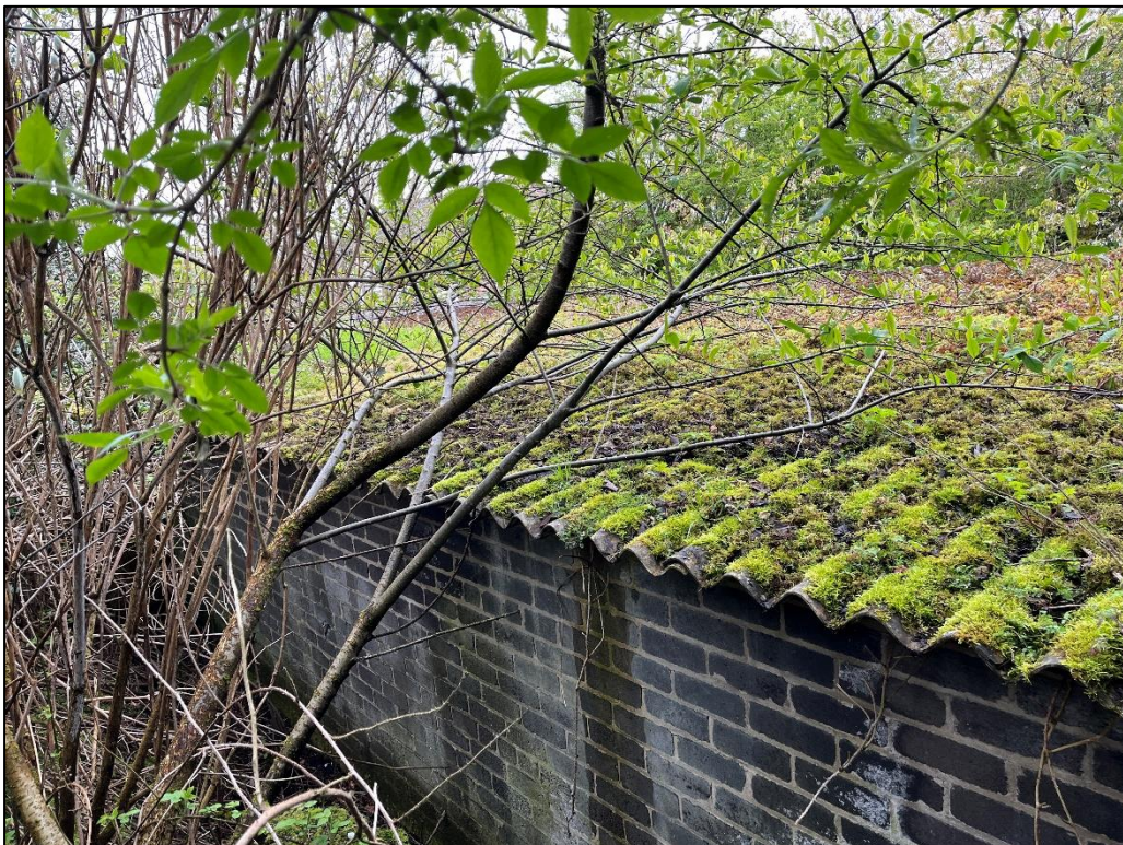
Plate 2 – Roof of B1 as seen from rear
