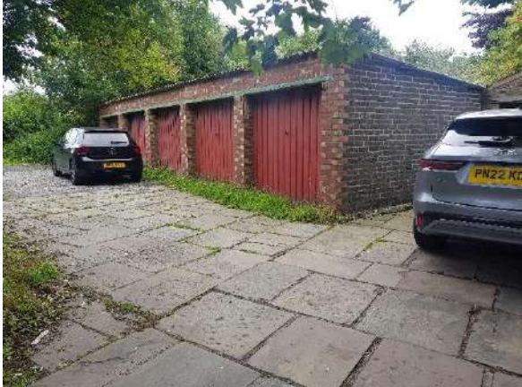
P4: Garages and driveway in the north of the site. Photo facing east.
