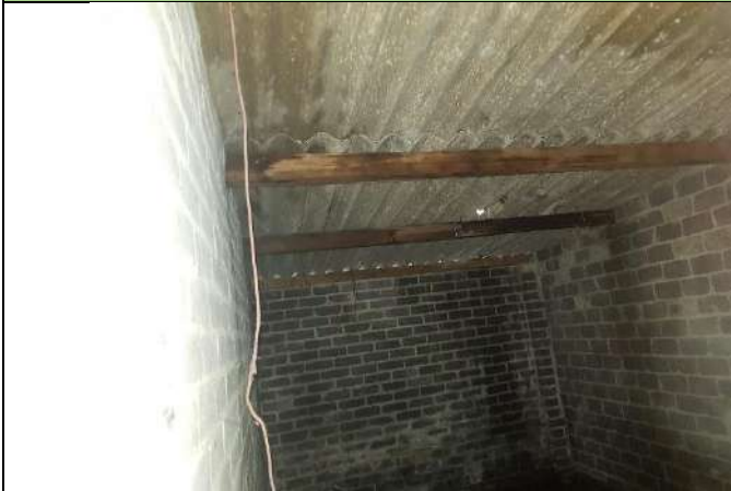
P5: View inside one of the garages located in the north of the site.
