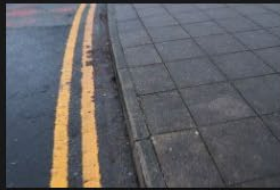
2A-2B – Rectory Lane – Kerbs and Footpath - 18-01-2026 (104)
