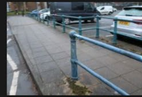
2A-2B – Rectory Lane – Kerbs and Footpath - 18-01-2026 (83)
