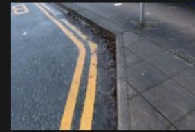
2A-2B – Rectory Lane – Kerbs and Footpath - 18-01-2026 (29)
