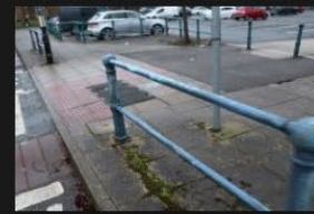
2A-2B – Rectory Lane – Kerbs and Footpath - 18-01-2026 (71)
