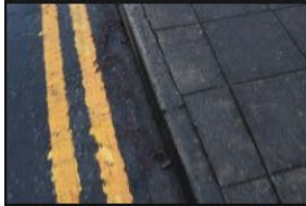
2A-2B – Rectory Lane – Kerbs and Footpath - 18-01-2026 (103)
