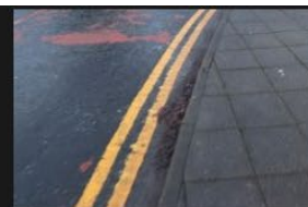
2A-2B - Rectory Lane - Kerbs and Footpath - 18-01-2026 (113)
