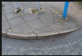
2A-2B – Rectory Lane – Kerbs and Footpath - 18-01-2026 (68)
