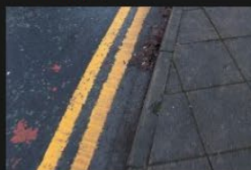
2A-2B - Rectory Lane - Kerbs and Footpath - 18-01-2026 (117)
