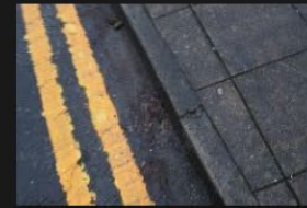
2A-2B – Rectory Lane – Kerbs and Footpath - 18-01-2026 (102)
