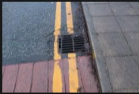
2A-2B – Rectory Lane – Kerbs and Footpath - 18-01-2026 (26)
