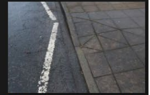
2A-2B – Rectory Lane – Kerbs and Footpath - 18-01-2026 (90)
