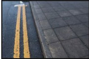
2A-2B – Rectory Lane – Kerbs and Footpath - 18-01-2026 (49)
