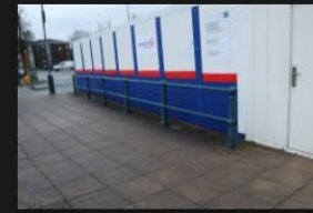
2A-2B – Rectory Lane – Kerbs and Footpath - 18-01-2026 (41)
