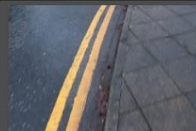
2A-2B - Rectory Lane - Kerbs and Footpath - 18-01-2026 (119)
