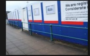
2A-2B – Rectory Lane – Kerbs and Footpath - 18-01-2026 (36)
