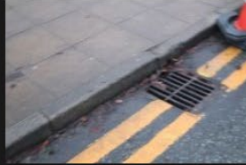
2A-2B – Rectory Lane – Kerbs and Footpath - 18-01-2026 (3)
