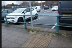
2A-2B – Rectory Lane – Kerbs and Footpath - 18-01-2026 (92)
