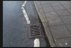
2A-2B – Rectory Lane – Kerbs and Footpath - 18-01-2026 (88)
