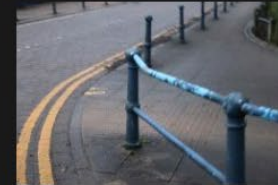
2A-2B – Rectory Lane – Kerbs and Footpath - 18-01-2026 (11)
