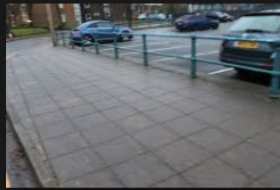
2A-2B – Rectory Lane – Kerbs and Footpath - 18-01-2026 (98)
