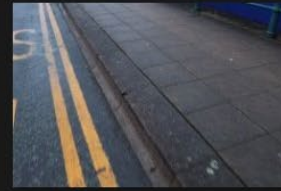
2A-2B – Rectory Lane – Kerbs and Footpath - 18-01-2026 (34)
