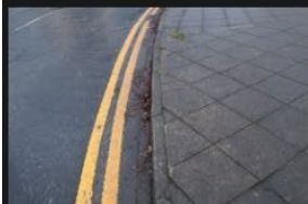
2A-2B - Rectory Lane - Kerbs and Footpath - 18-01-2026 (121)
