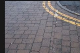
2A-2B – Rectory Lane – Kerbs and Footpath - 18-01-2026 (17)
