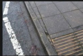
2A-2B – Rectory Lane – Kerbs and Footpath - 18-01-2026 (94)
