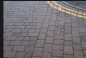
2A-2B – Rectory Lane – Kerbs and Footpath - 18-01-2026 (16)
