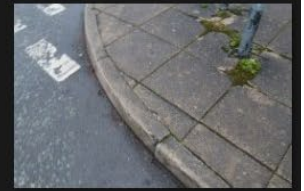
2A-2B – Rectory Lane – Kerbs and Footpath - 18-01-2026 (54)
