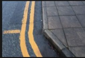
2A-2B – Rectory Lane – Kerbs and Footpath - 18-01-2026 (45)
