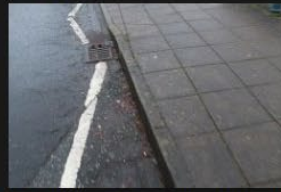
2A-2B – Rectory Lane – Kerbs and Footpath - 18-01-2026 (87)
