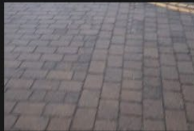
2A-2B – Rectory Lane – Kerbs and Footpath - 18-01-2026 (15)
