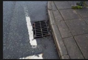
2A-2B – Rectory Lane – Kerbs and Footpath - 18-01-2026 (52)
