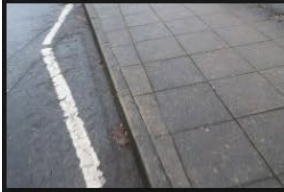
2A-2B – Rectory Lane – Kerbs and Footpath - 18-01-2026 (85)
