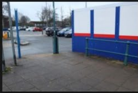
2A-2B – Rectory Lane – Kerbs and Footpath - 18-01-2026 (50)
