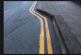
2A-2B – Rectory Lane – Kerbs and Footpath - 18-01-2026 (40)
