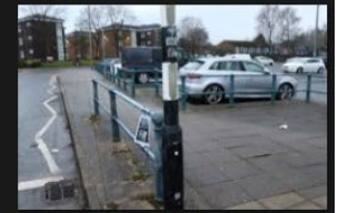
2A-2B – Rectory Lane – Kerbs and Footpath - 18-01-2026 (78)
