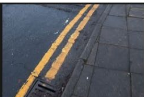
2A-2B - Rectory Lane - Kerbs and Footpath - 18-01-2026 (110)
