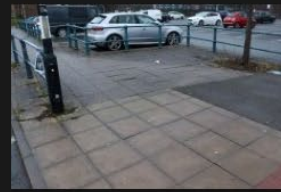
2A-2B – Rectory Lane – Kerbs and Footpath - 18-01-2026 (76)
