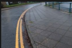
2A-2B - Rectory Lane - Kerbs and Footpath - 18-01-2026 (122)
