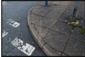
2A-2B – Rectory Lane – Kerbs and Footpath - 18-01-2026 (55)
