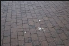
2A-2B – Rectory Lane – Kerbs and Footpath - 18-01-2026 (14)
