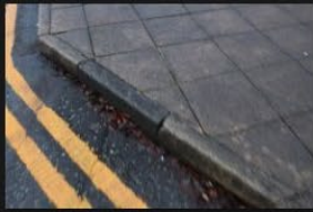
2A-2B – Rectory Lane – Kerbs and Footpath - 18-01-2026 (44)
