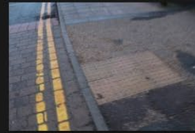
2A-2B – Rectory Lane – Kerbs and Footpath - 18-01-2026 (22)
