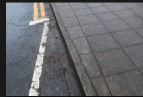
2A-2B – Rectory Lane – Kerbs and Footpath - 18-01-2026 (95)
