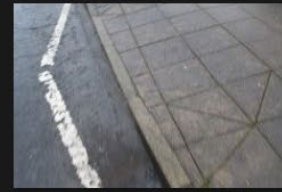
2A-2B – Rectory Lane – Kerbs and Footpath - 18-01-2026 (89)
