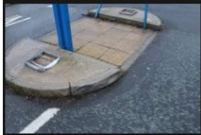
2A-2B – Rectory Lane – Kerbs and Footpath - 18-01-2026 (61)
