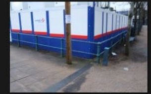
2A-2B – Rectory Lane – Kerbs and Footpath - 18-01-2026 (24)
