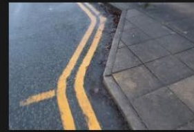
2A-2B – Rectory Lane – Kerbs and Footpath - 18-01-2026 (28)
