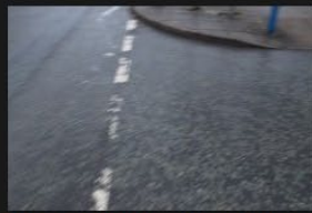
2A-2B – Rectory Lane – Kerbs and Footpath - 18-01-2026 (63)
