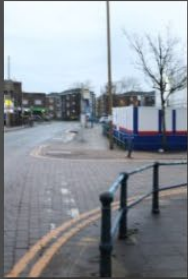
2A-2B – Rectory Lane – Kerbs and Footpath - 18-01-2026 (1)
