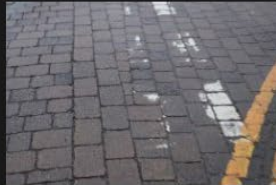
2A-2B – Rectory Lane – Kerbs and Footpath - 18-01-2026 (9)
