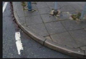
2A-2B – Rectory Lane – Kerbs and Footpath - 18-01-2026 (69)
