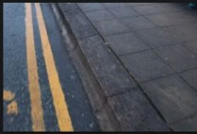
2A-2B – Rectory Lane – Kerbs and Footpath - 18-01-2026 (38)
