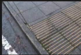
2A-2B – Rectory Lane – Kerbs and Footpath - 18-01-2026 (93)
