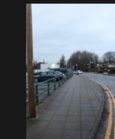
2A-2B - Rectory Lane - Kerbs and Footpath - 18-01-2026 (123)
