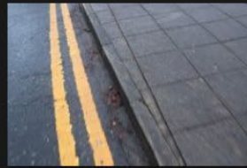
2A-2B – Rectory Lane – Kerbs and Footpath - 18-01-2026 (100)
