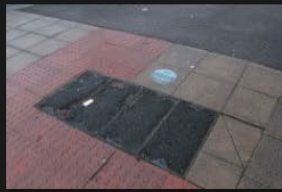
2A-2B – Rectory Lane – Kerbs and Footpath - 18-01-2026 (74)
