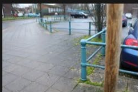
2A-2B - Rectory Lane - Kerbs and Footpath - 18-01-2026 (116)
