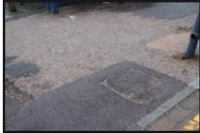
2A-2B – Rectory Lane – Kerbs and Footpath - 18-01-2026 (19)
