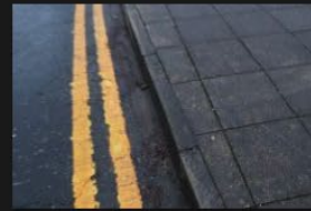
2A-2B – Rectory Lane – Kerbs and Footpath - 18-01-2026 (101)
