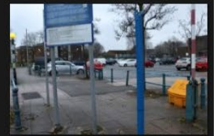
2A-2B – Rectory Lane – Kerbs and Footpath - 18-01-2026 (66)
