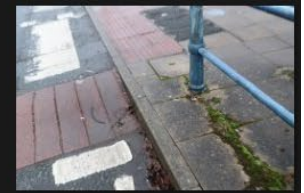
2A-2B – Rectory Lane – Kerbs and Footpath - 18-01-2026 (72)
