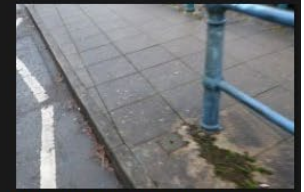
2A-2B – Rectory Lane – Kerbs and Footpath - 18-01-2026 (84)
