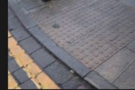
2A-2B – Rectory Lane – Kerbs and Footpath - 18-01-2026 (5)
