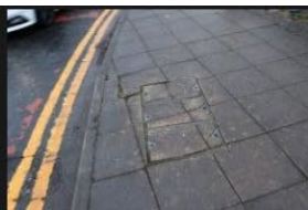
2A-2B - Rectory Lane - Kerbs and Footpath - 18-01-2026 (111)
