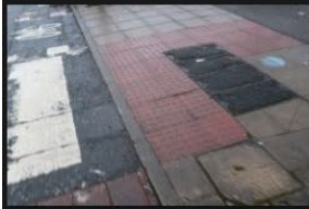
2A-2B – Rectory Lane – Kerbs and Footpath - 18-01-2026 (73)
