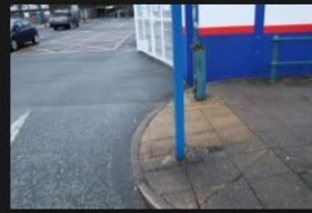
2A-2B – Rectory Lane – Kerbs and Footpath - 18-01-2026 (58)
