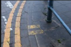
2A-2B – Rectory Lane – Kerbs and Footpath - 18-01-2026 (8)
