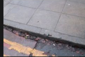
2A-2B – Rectory Lane – Kerbs and Footpath - 18-01-2026 (4)
