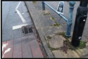
2A-2B – Rectory Lane – Kerbs and Footpath - 18-01-2026 (79)
