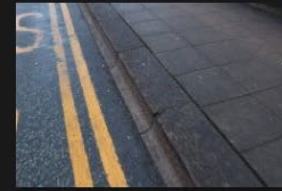
2A-2B – Rectory Lane – Kerbs and Footpath - 18-01-2026 (35)
