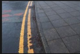
2A-2B – Rectory Lane – Kerbs and Footpath - 18-01-2026 (105)
