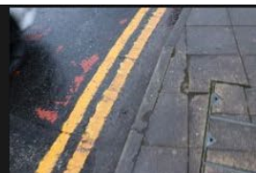
2A-2B - Rectory Lane - Kerbs and Footpath - 18-01-2026 (112)
