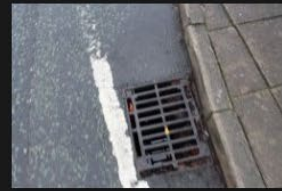
2A-2B – Rectory Lane – Kerbs and Footpath - 18-01-2026 (53)
