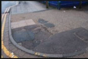
2A-2B – Rectory Lane – Kerbs and Footpath - 18-01-2026 (20)
