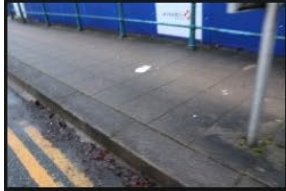
2A-2B – Rectory Lane – Kerbs and Footpath - 18-01-2026 (31)
