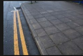
2A-2B – Rectory Lane – Kerbs and Footpath - 18-01-2026 (47)
