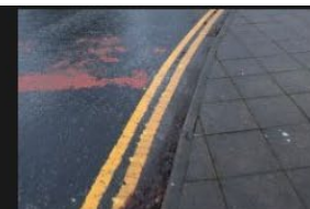
2A-2B - Rectory Lane - Kerbs and Footpath - 18-01-2026 (114)
