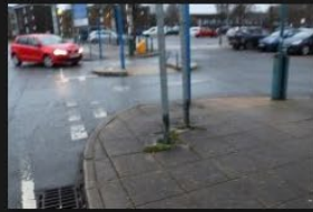
2A-2B – Rectory Lane – Kerbs and Footpath - 18-01-2026 (51)
