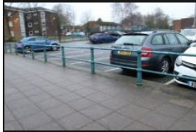
2A-2B – Rectory Lane – Kerbs and Footpath - 18-01-2026 (97)
