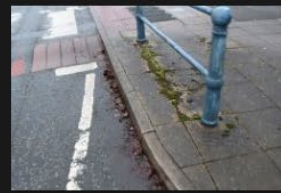
2A-2B – Rectory Lane – Kerbs and Footpath - 18-01-2026 (70)
