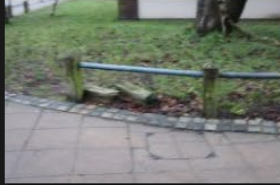
2A-2B – Rectory Lane – Kerbs and Footpath - 18-01-2026 (2)
