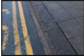
2A-2B – Rectory Lane – Kerbs and Footpath - 18-01-2026 (37)
