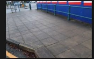
2A-2B – Rectory Lane – Kerbs and Footpath - 18-01-2026 (42)
