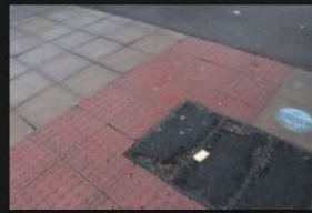
2A-2B – Rectory Lane – Kerbs and Footpath - 18-01-2026 (75)
