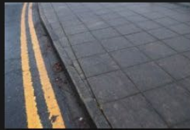
2A-2B – Rectory Lane – Kerbs and Footpath - 18-01-2026 (99)
