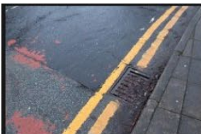
2A-2B - Rectory Lane - Kerbs and Footpath - 18-01-2026 (109)
