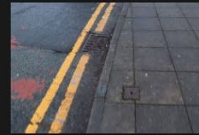
2A-2B – Rectory Lane – Kerbs and Footpath - 18-01-2026 (108)
