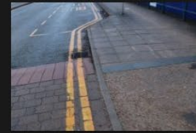
2A-2B – Rectory Lane – Kerbs and Footpath - 18-01-2026 (23)
