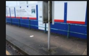
2A-2B – Rectory Lane – Kerbs and Footpath - 18-01-2026 (30)
