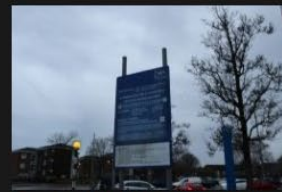
2A-2B – Rectory Lane – Kerbs and Footpath - 18-01-2026 (65)
