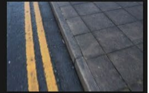
2A-2B – Rectory Lane – Kerbs and Footpath - 18-01-2026 (48)
