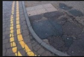
2A-2B – Rectory Lane – Kerbs and Footpath - 18-01-2026 (21)
