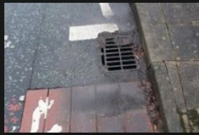
2A-2B – Rectory Lane – Kerbs and Footpath - 18-01-2026 (80)
