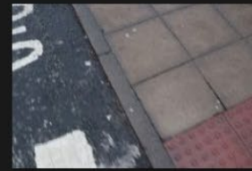
2A-2B – Rectory Lane – Kerbs and Footpath - 18-01-2026 (77)
