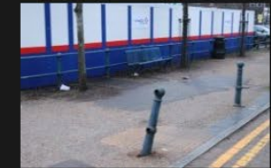
2A-2B – Rectory Lane – Kerbs and Footpath - 18-01-2026 (18)
