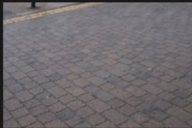
2A-2B – Rectory Lane – Kerbs and Footpath - 18-01-2026 (13)
