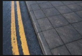
2A-2B – Rectory Lane – Kerbs and Footpath - 18-01-2026 (46)
