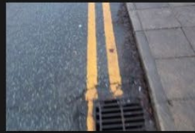
2A-2B – Rectory Lane – Kerbs and Footpath - 18-01-2026 (27)
