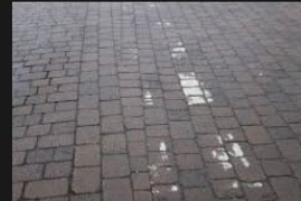
2A-2B – Rectory Lane – Kerbs and Footpath - 18-01-2026 (10)
