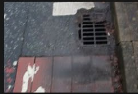
2A-2B – Rectory Lane – Kerbs and Footpath - 18-01-2026 (81)
