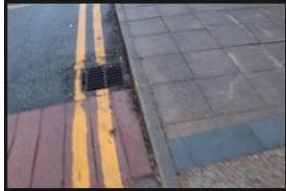
2A-2B – Rectory Lane – Kerbs and Footpath - 18-01-2026 (25)
