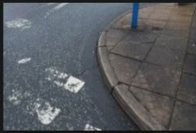
2A-2B – Rectory Lane – Kerbs and Footpath - 18-01-2026 (56)
