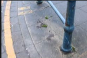
2A-2B – Rectory Lane – Kerbs and Footpath - 18-01-2026 (7)
