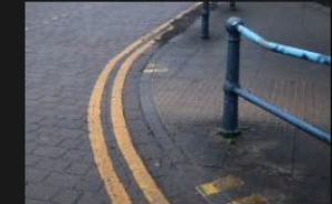
2A-2B – Rectory Lane – Kerbs and Footpath - 18-01-2026 (12)
