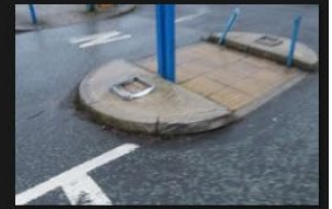
2A-2B – Rectory Lane – Kerbs and Footpath - 18-01-2026 (60)
