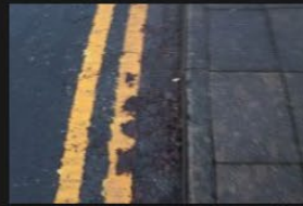
2A-2B – Rectory Lane – Kerbs and Footpath - 18-01-2026 (106)
