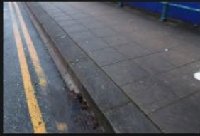
2A-2B – Rectory Lane – Kerbs and Footpath - 18-01-2026 (32)
