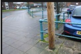
2A-2B - Rectory Lane - Kerbs and Footpath - 18-01-2026 (115)
