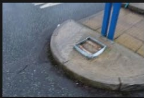
2A-2B – Rectory Lane – Kerbs and Footpath - 18-01-2026 (62)
