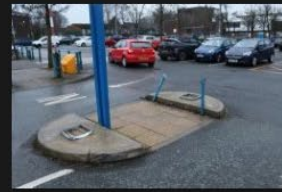
2A-2B – Rectory Lane – Kerbs and Footpath - 18-01-2026 (59)
