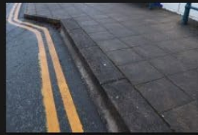
2A-2B – Rectory Lane – Kerbs and Footpath - 18-01-2026 (39)
