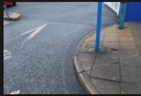
2A-2B – Rectory Lane – Kerbs and Footpath - 18-01-2026 (57)
