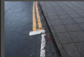
2A-2B – Rectory Lane – Kerbs and Footpath - 18-01-2026 (96)
