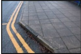
2A-2B – Rectory Lane – Kerbs and Footpath - 18-01-2026 (43)
