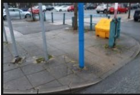
2A-2B – Rectory Lane – Kerbs and Footpath - 18-01-2026 (67)
