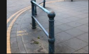
2A-2B – Rectory Lane – Kerbs and Footpath - 18-01-2026 (6)
