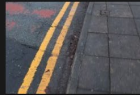
2A-2B – Rectory Lane – Kerbs and Footpath - 18-01-2026 (107)
