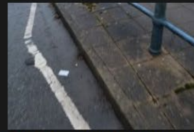
2A-2B – Rectory Lane – Kerbs and Footpath - 18-01-2026 (82)
