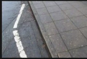
2A-2B – Rectory Lane – Kerbs and Footpath - 18-01-2026 (86)
