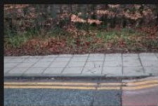
1A-1B - Rectory Lane - Road Surface - 18-01-2026 (51)
