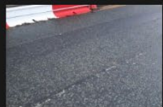
1A-1B - Rectory Lane - Road Surface - 18-01-2026 (39)
