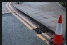
1A-1B - Rectory Lane - Road Surface - 18-01-2026 (43)
