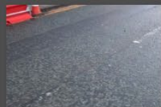
1A-1B - Rectory Lane - Road Surface - 18-01-2026 (40)
