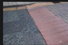
1A-1B - Rectory Lane - Road Surface - 18-01-2026 (48)
