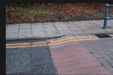
1A-1B - Rectory Lane - Road Surface - 18-01-2026 (49)
