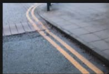
1A-1B - Rectory Lane - Road Surface - 18-01-2026 (44)
