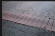
1A-1B - Rectory Lane - Road Surface - 18-01-2026 (46)
