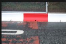
1A-1B - Rectory Lane - Road Surface - 18-01-2026 (37)
