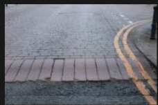
1A-1B - Rectory Lane - Road Surface - 18-01-2026 (45)
