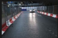
1A-1B - Rectory Lane - Road Surface - 18-01-2026 (52)
