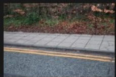
1A-1B - Rectory Lane - Road Surface - 18-01-2026 (50)
