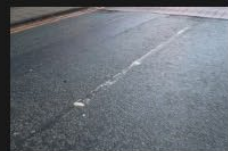
1A-1B - Rectory Lane - Road Surface - 18-01-2026 (41)
