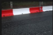
1A-1B - Rectory Lane - Road Surface - 18-01-2026 (38)
