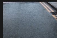
1A-1B - Rectory Lane - Road Surface - 18-01-2026 (42)
