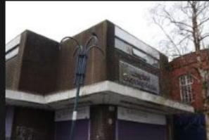
☁ 15A-15B – Pedestrian Footpath - 18-01-2026 (51)
