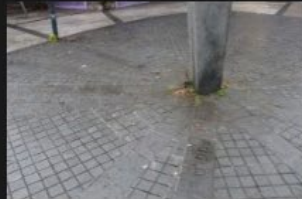
☁ 15A-15B – Pedestrian Footpath - 18-01-2026 (50)
