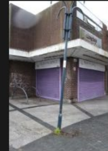
☁ 15A-15B – Pedestrian Footpath - 18-01-2026 (53)
