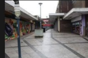
☁ 15A-15B – Pedestrian Footpath - 18-01-2026 (52)
