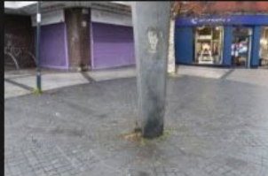
☁ 15A-15B – Pedestrian Footpath - 18-01-2026 (49)
