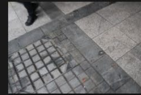
14A-14B - Pedestrian Footpath - 18-01-2026 (53)
