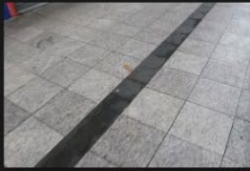
14A-14B – Pedestrian Footpath - 18-01-2026 (38)
