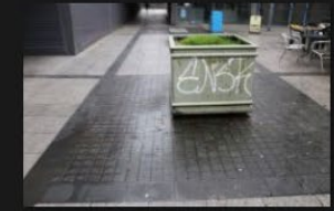
14A-14B – Pedestrian Footpath - 18-01-2026 (42)
