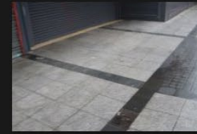
14A-14B – Pedestrian Footpath - 18-01-2026 (41)
