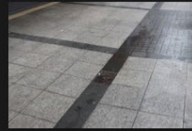
14A-14B – Pedestrian Footpath - 18-01-2026 (40)
