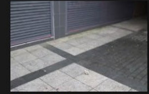
14A-14B – Pedestrian Footpath - 18-01-2026 (48)
