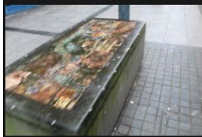
14A-14B – Pedestrian Footpath - 18-01-2026 (25)
