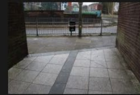
14A-14B - Pedestrian Footpath - 18-01-2026 (59)
