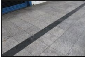
14A-14B – Pedestrian Footpath - 18-01-2026 (31)
