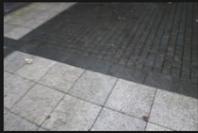
14A-14B - Pedestrian Footpath - 18-01-2026 (49)
