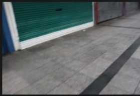
14A-14B – Pedestrian Footpath - 18-01-2026 (32)
