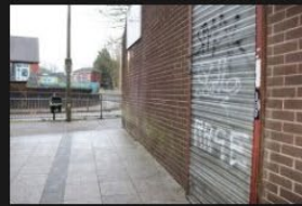
14A-14B - Pedestrian Footpath - 18-01-2026 (57)
