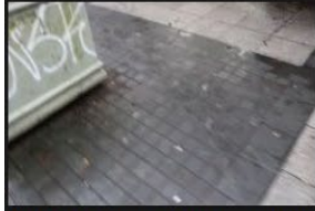
14A-14B – Pedestrian Footpath - 18-01-2026 (43)
