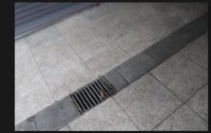
14A-14B - Pedestrian Footpath - 18-01-2026 (54)
