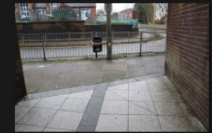
14A-14B - Pedestrian Footpath - 18-01-2026 (60)
