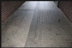
14A-14B - Pedestrian Footpath - 18-01-2026 (55)
