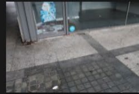
14A-14B - Pedestrian Footpath - 18-01-2026 (52)
