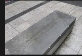
14A-14B – Pedestrian Footpath - 18-01-2026 (47)
