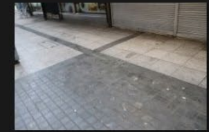
14A-14B – Pedestrian Footpath - 18-01-2026 (36)
