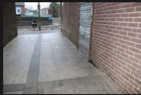
14A-14B - Pedestrian Footpath - 18-01-2026 (56)
