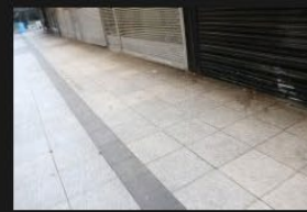
14A-14B – Pedestrian Footpath - 18-01-2026 (28)
