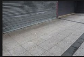
14A-14B – Pedestrian Footpath - 18-01-2026 (39)
