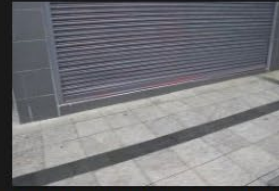
14A-14B – Pedestrian Footpath - 18-01-2026 (46)
