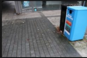
14A-14B - Pedestrian Footpath - 18-01-2026 (50)
