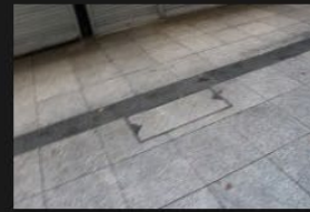
14A-14B – Pedestrian Footpath - 18-01-2026 (34)
