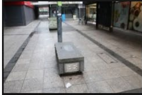
14A-14B – Pedestrian Footpath - 18-01-2026 (37)
