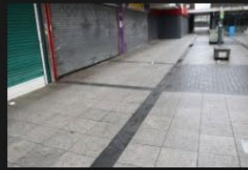
14A-14B – Pedestrian Footpath - 18-01-2026 (33)
