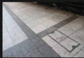
14A-14B – Pedestrian Footpath - 18-01-2026 (27)
