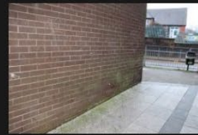
14A-14B - Pedestrian Footpath - 18-01-2026 (58)
