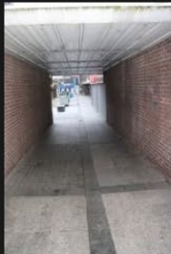
14A-14B - Pedestrian Footpath - 18-01-2026 (61)
