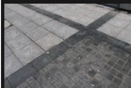
12A-12B – Pedestrian Footpath - 18-01-2026 (19)
