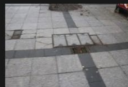
12A-12B – Pedestrian Footpath - 18-01-2026 (11)
