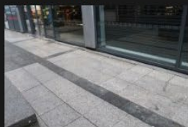
12A-12B – Pedestrian Footpath - 18-01-2026 (20)
