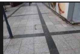
12A-12B – Pedestrian Footpath - 18-01-2026 (5)
