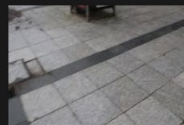
12A-12B – Pedestrian Footpath - 18-01-2026 (12)
