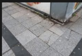
12A-12B – Pedestrian Footpath - 18-01-2026 (8)
