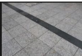
12A-12B – Pedestrian Footpath - 18-01-2026 (3)
