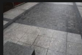
12A-12B – Pedestrian Footpath - 18-01-2026 (23)
