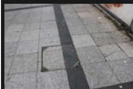
12A-12B – Pedestrian Footpath - 18-01-2026 (7)
