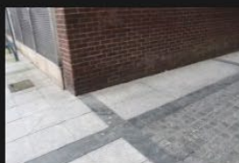
12A-12B – Pedestrian Footpath - 18-01-2026 (15)
