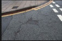
10A-10B – Access Road – Road Surface - 18-01-2026 (8)
