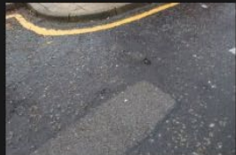
10A-10B - Access Road - Road Surface - 18-01-2026 (37)
