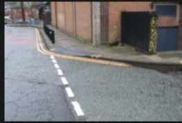
10A-10B – Access Road – Road Surface - 18-01-2026 (2)
