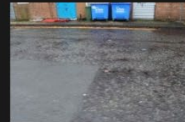
10A-10B - Access Road - Road Surface - 18-01-2026 (47)
