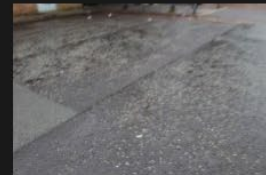
10A-10B - Access Road - Road Surface - 18-01-2026 (45)
