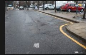
10A-10B - Access Road - Road Surface - 18-01-2026 (30)
