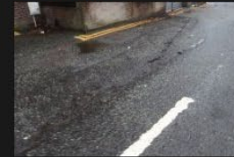
10A-10B – Access Road – Road Surface - 18-01-2026 (17)
