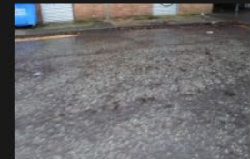
10A-10B - Access Road - Road Surface - 18-01-2026 (48)
