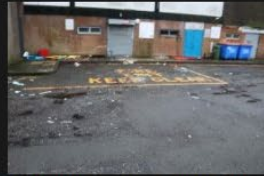
10A-10B - Access Road - Road Surface - 18-01-2026 (32)
