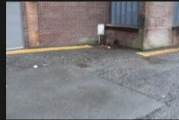
10A-10B – Access Road – Road Surface - 18-01-2026 (15)
