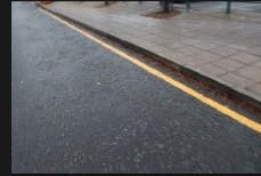
10A-10B – Access Road – Road Surface - 18-01-2026 (10)
