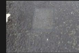
10A-10B – Access Road – Road Surface - 18-01-2026 (18)
