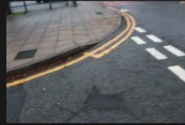
10A-10B – Access Road – Road Surface - 18-01-2026 (9)
