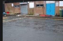
10A-10B - Access Road - Road Surface - 18-01-2026 (46)
