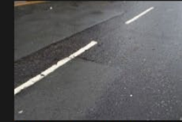
10A-10B – Access Road – Road Surface - 18-01-2026 (12)
