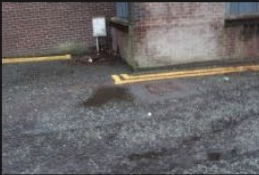
10A-10B – Access Road – Road Surface - 18-01-2026 (19)
