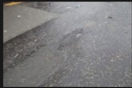
10A-10B - Access Road - Road Surface - 18-01-2026 (25)
