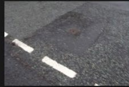
10A-10B – Access Road – Road Surface - 18-01-2026 (3)
