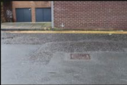
10A-10B – Access Road – Road Surface - 18-01-2026 (13)
