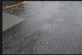
10A-10B - Access Road - Road Surface - 18-01-2026 (26)
