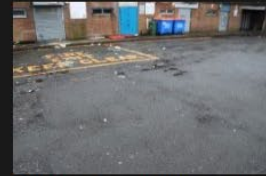
10A-10B - Access Road - Road Surface - 18-01-2026 (33)
