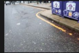
10A-10B - Access Road - Road Surface - 18-01-2026 (29)
