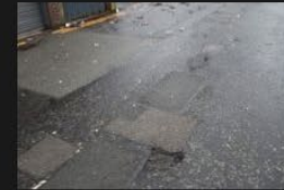
10A-10B – Access Road – Road Surface - 18-01-2026 (23)
