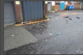
10A-10B - Access Road - Road Surface - 18-01-2026 (27)
