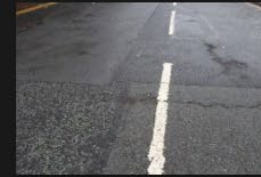
10A-10B – Access Road – Road Surface - 18-01-2026 (5)
