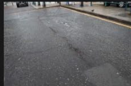
10A-10B - Access Road - Road Surface - 18-01-2026 (44)
