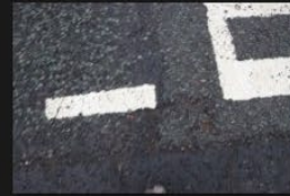
10A-10B – Access Road – Road Surface - 18-01-2026 (4)
