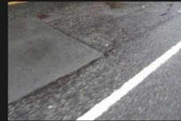
10A-10B – Access Road – Road Surface - 18-01-2026 (16)
