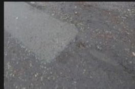
10A-10B - Access Road - Road Surface - 18-01-2026 (38)
