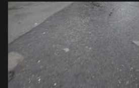
10A-10B - Access Road - Road Surface - 18-01-2026 (42)
