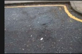
10A-10B - Access Road - Road Surface - 18-01-2026 (35)
