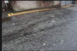
10A-10B – Access Road – Road Surface - 18-01-2026 (20)
