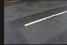
10A-10B – Access Road – Road Surface - 18-01-2026 (11)
