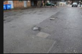
10A-10B - Access Road - Road Surface - 18-01-2026 (34)
