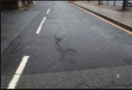
10A-10B – Access Road – Road Surface - 18-01-2026 (7)
