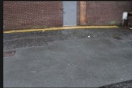
10A-10B – Access Road – Road Surface - 18-01-2026 (14)
