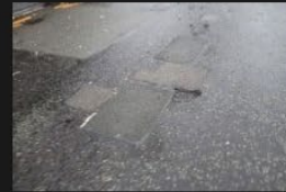
10A-10B – Access Road – Road Surface - 18-01-2026 (22)
