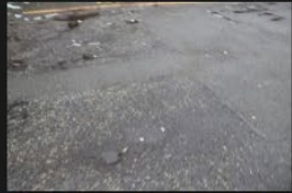
10A-10B - Access Road - Road Surface - 18-01-2026 (31)
