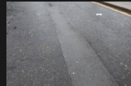
10A-10B - Access Road - Road Surface - 18-01-2026 (39)
