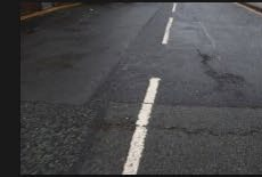
10A-10B – Access Road – Road Surface - 18-01-2026 (6)
