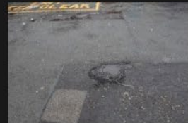
10A-10B - Access Road - Road Surface - 18-01-2026 (40)
