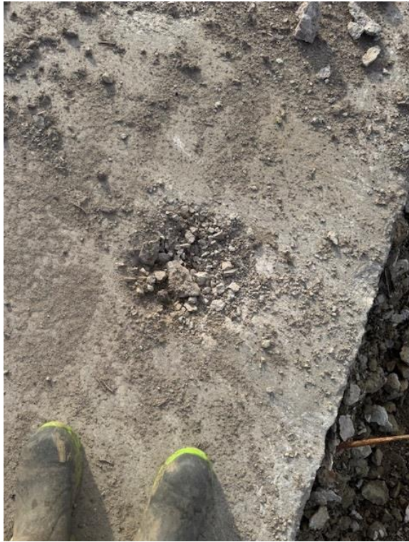
Area B – Concrete at surface
