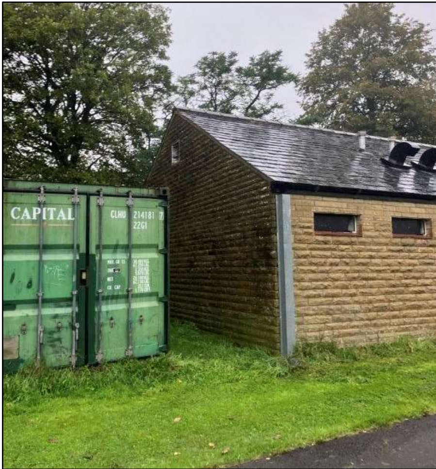
Figure 2-D: Photograph showing area of proposed pavilion extension.
