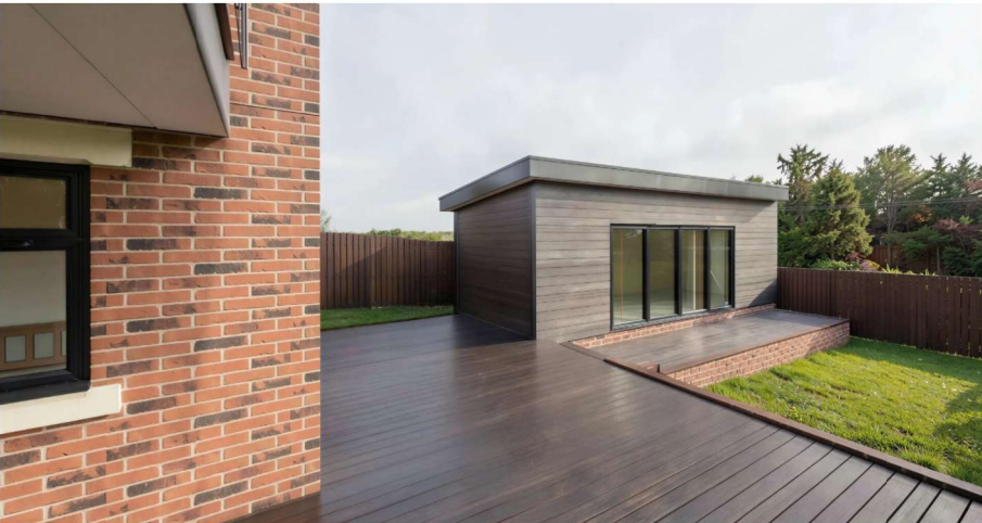
View of Outbuilding
