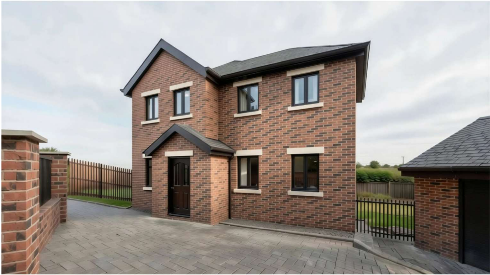
Front External View
