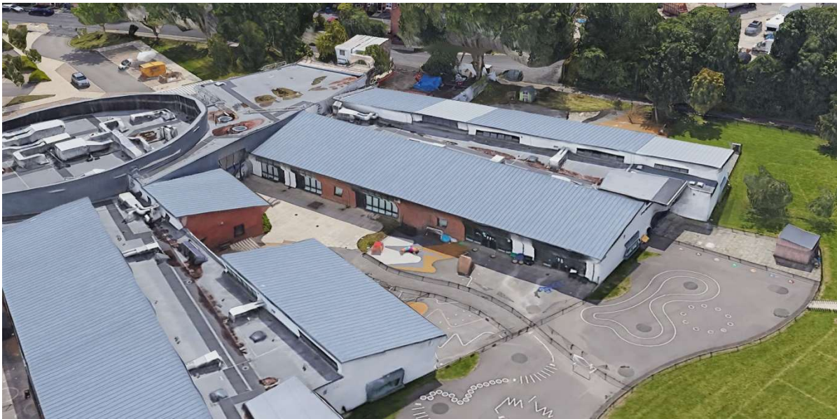
The existing school viewed from the north west.
