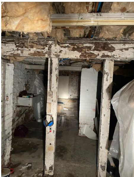
Photograph 3 – Cellar with removed ceiling
