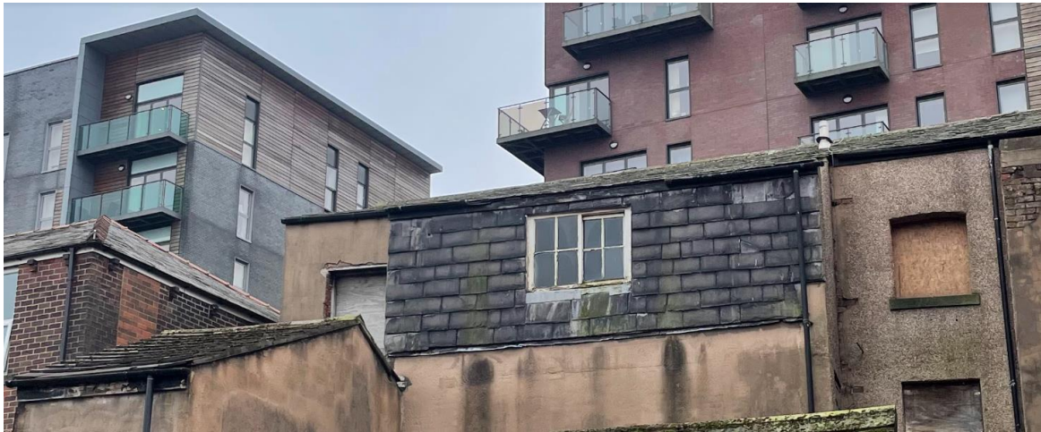
Photograph 16 – Third floor wall and second floor rooftop
