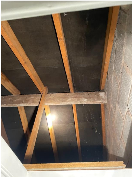
Photograph 5 – First floor loft void
