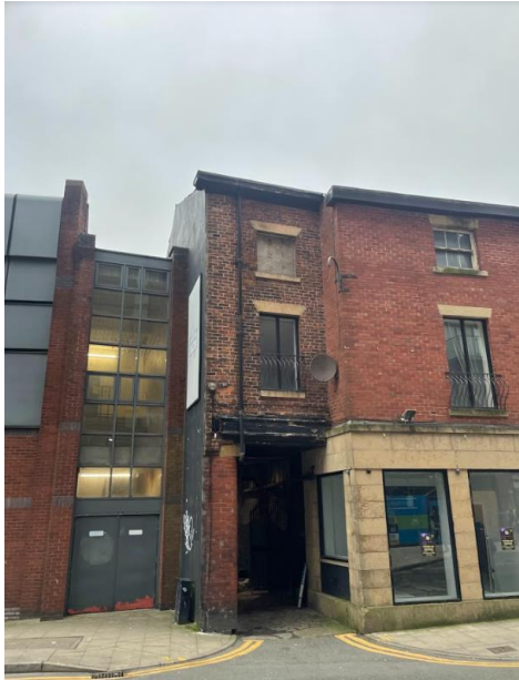
Photograph 9 – Southern aspect of B1
