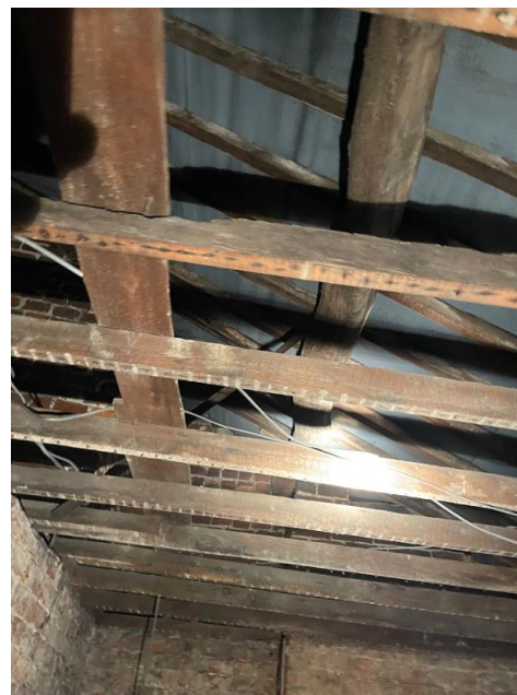
Photograph 8 – Beams present within second floor rooftop
