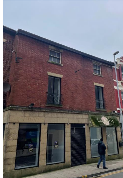
Photograph 10 – Southern aspect of B1
