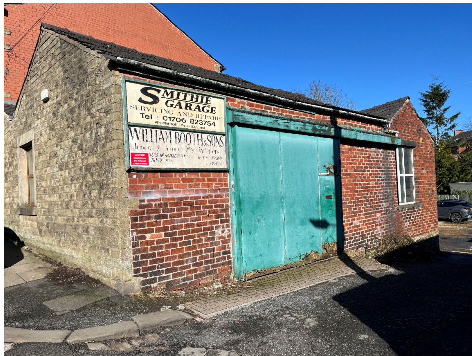
Existing garage viewed from Spring Street.
