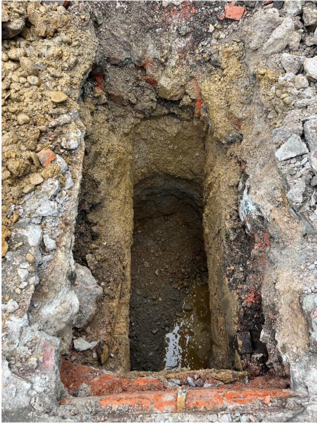
Station Works: 18/07/23 TP05 Complete
