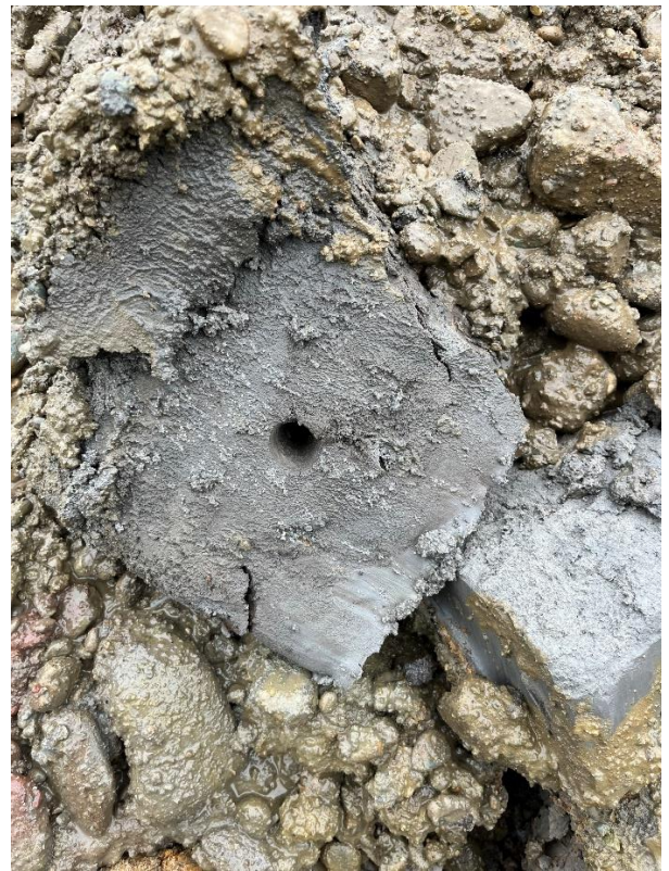
Station Works: 18/07/23 Soft Clay at 2.0m bgl
