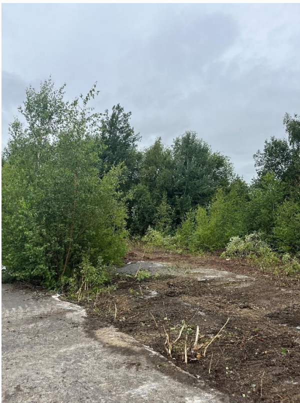
Station Works: 18/07/23 Veg Clearance (NW)
