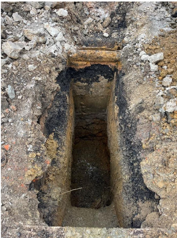
Station Works: 18/07/23 TP01 Complete
