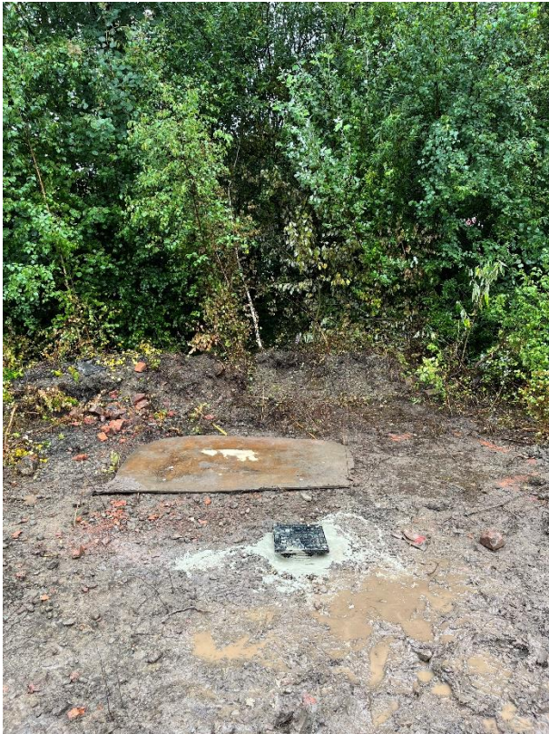
Station Works: 26/07/23 BH01A Install
