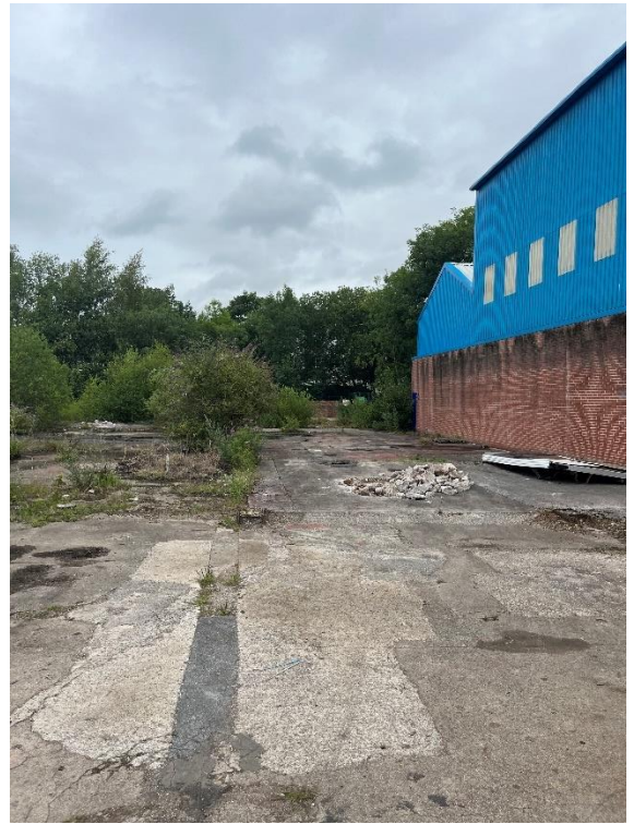
Station Works: 18/07/23 East Boundary
