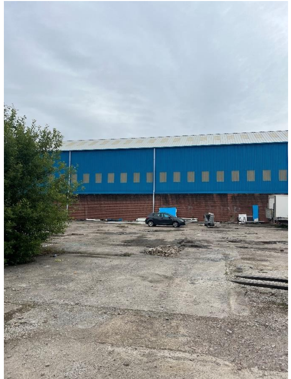
Station Works: 18/07/23 Site Photo East
