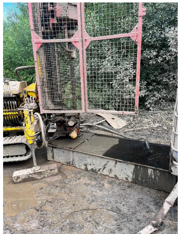
Station Works: 26/07/23 BH02 Rotary Water Flush Coal at 46.5m
