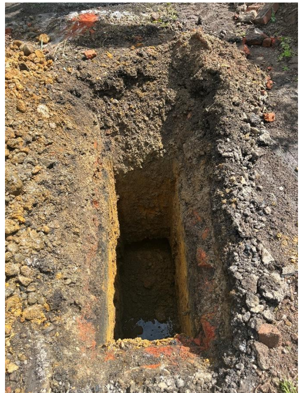
Station Works: 19/07/23 TP10 Complete
