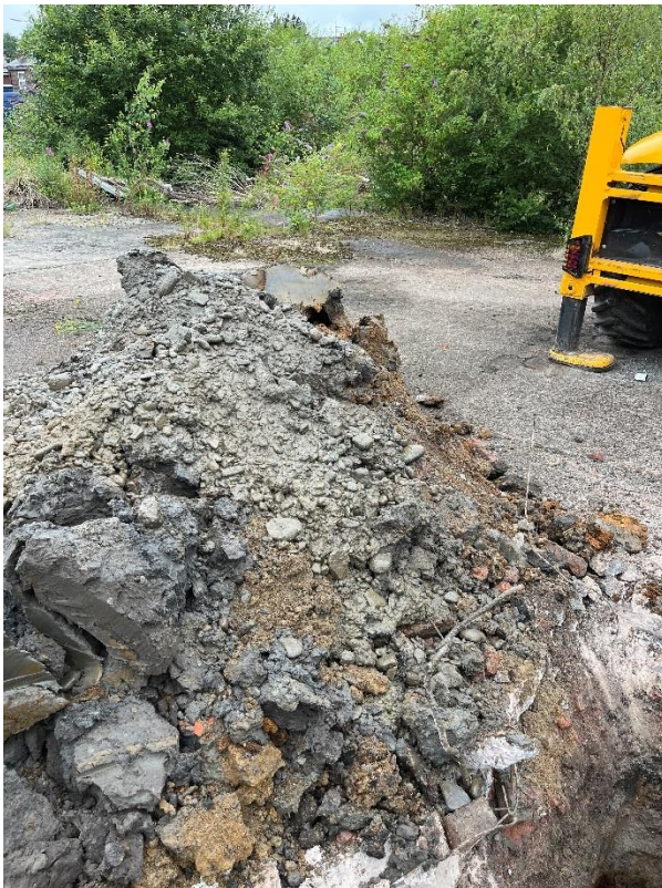
Station Works: 18/07/23 TP03 Arisings
