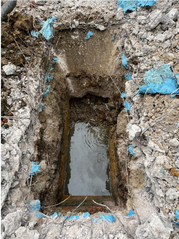
Station Works: 18/07/23 TP04 Complete
