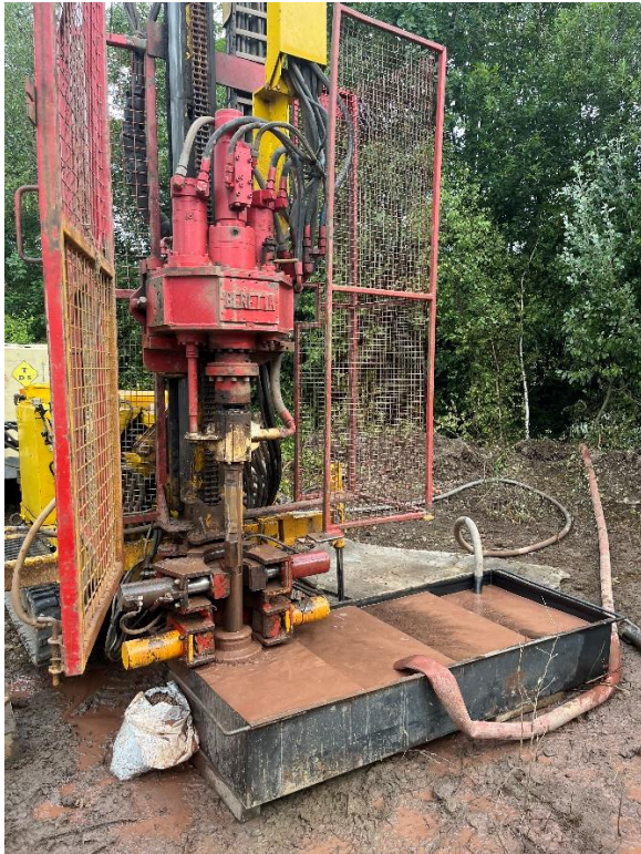
Station Works: 21/07/23 BH01A Rotary Water Flush
