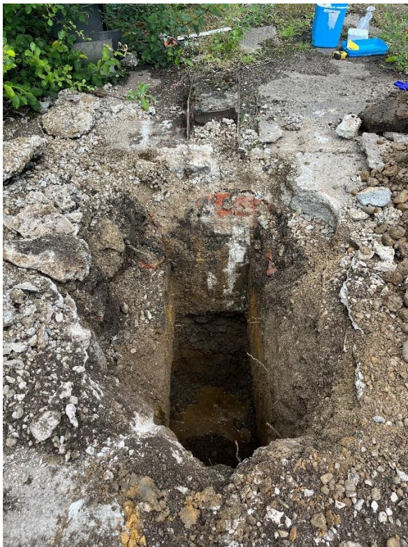
Station Works: 19/07/23 TP09 Pad Footing
