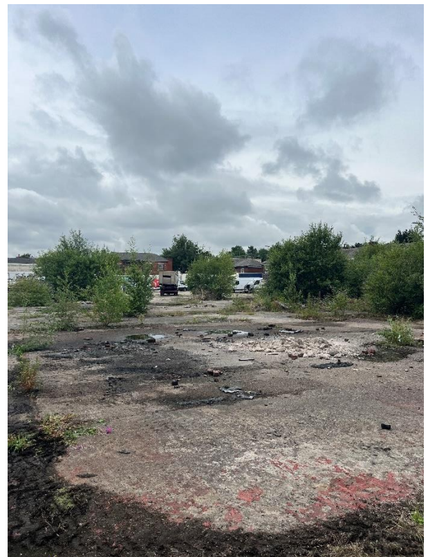
Station Works: 18/07/23 Site Photo South
