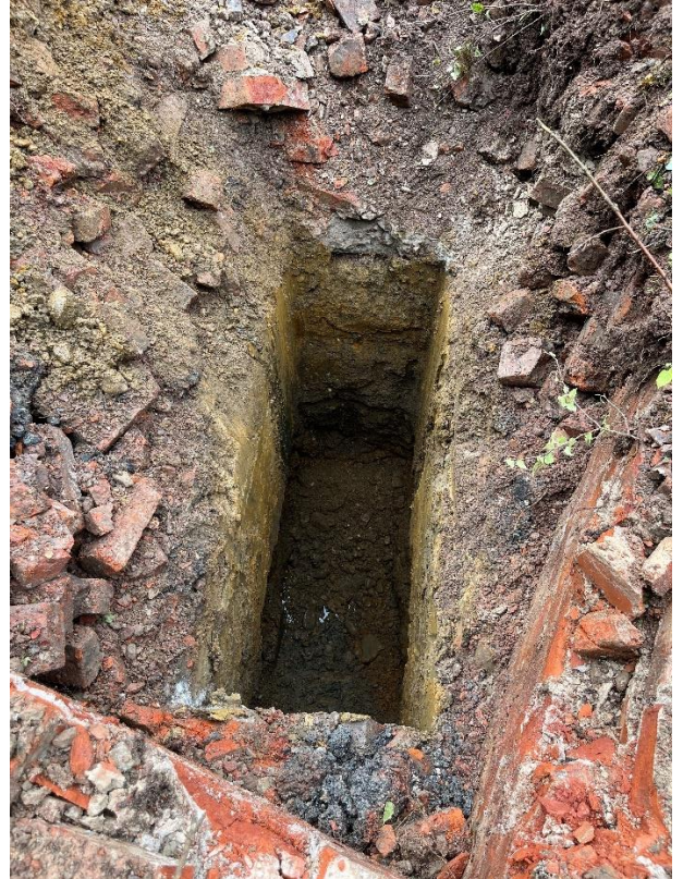
Station Works: 19/07/23 TP08 Complete
