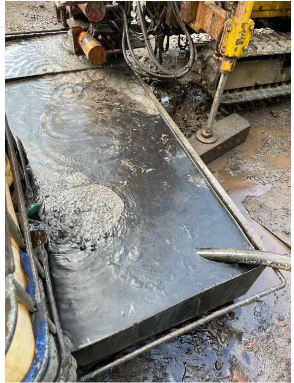
Station Works: 21/07/23 BH01A Rotary Water Flush Coal at 47.0m
