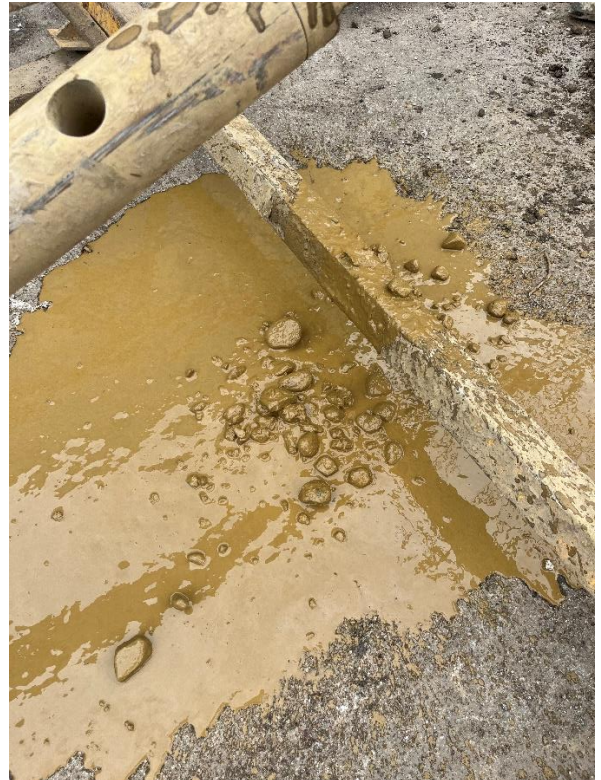
Station Works: 25/07/23 BH03 Natural Gravel 2.0m
