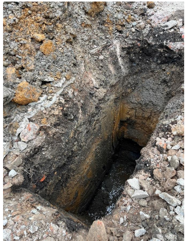
Station Works: 18/07/23 TP02 Side View
