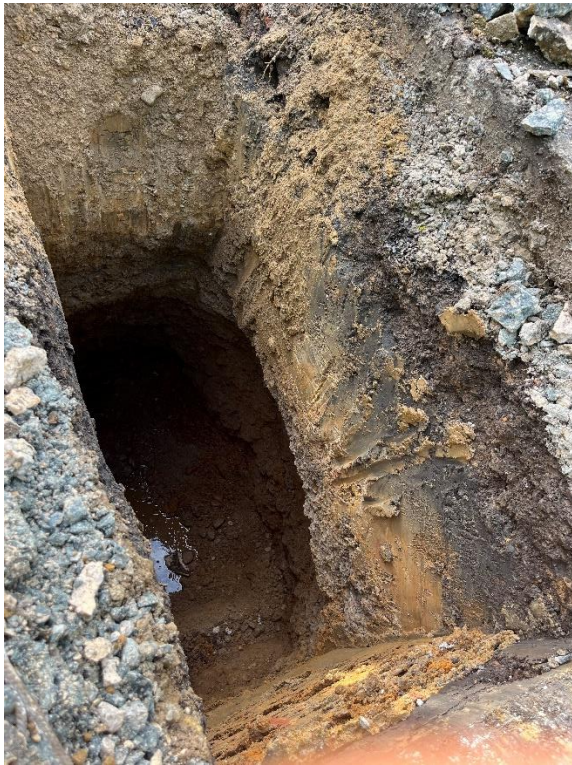
Station Works: 19/07/23 TP06 Side View
