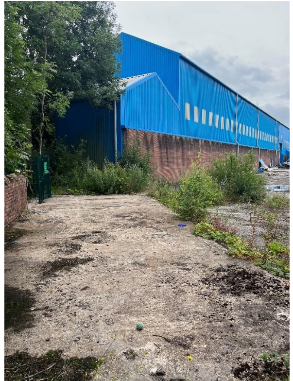
Station Works: 18/07/23 Concrete Plinth (NE)
