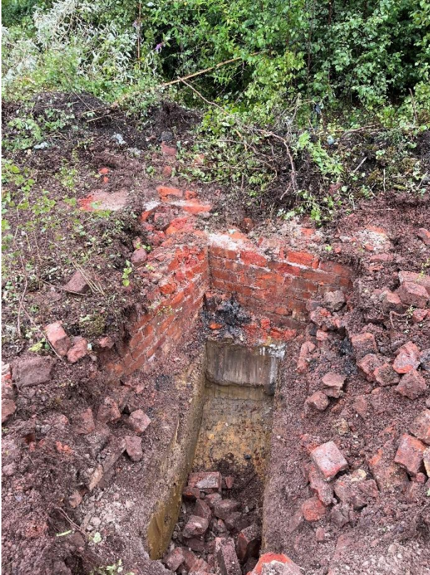
Station Works: 19/07/23 TP08 Buried Brick Wall
