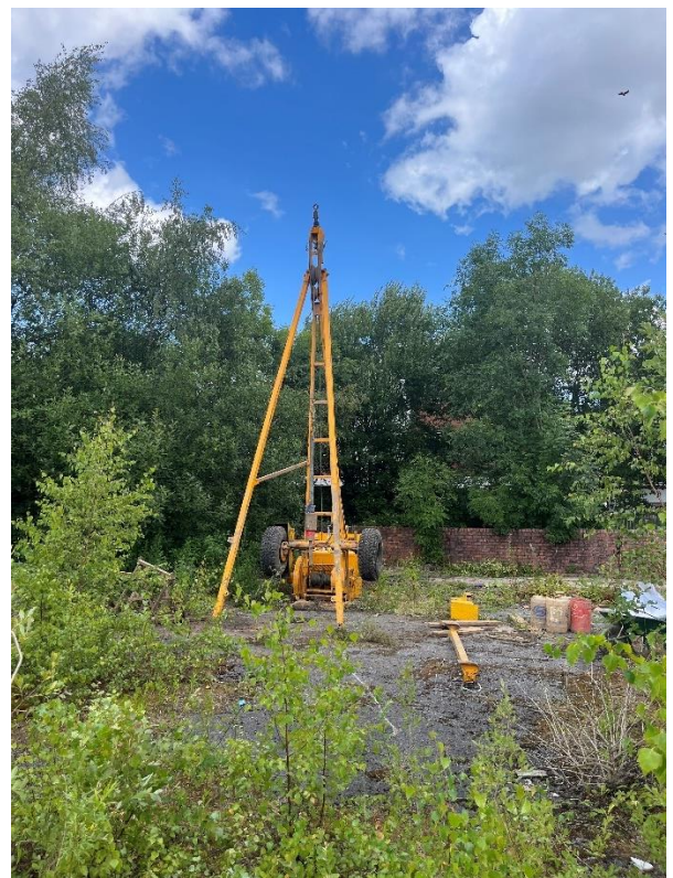
Station Works: 23/07/23 BH02 Location
