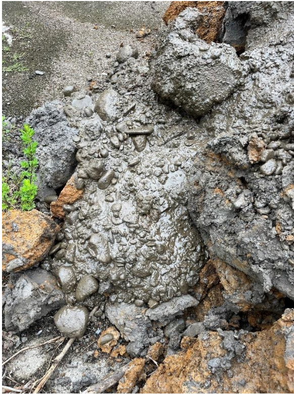
Station Works: 18/07/23 TP02 Oily Sheen
