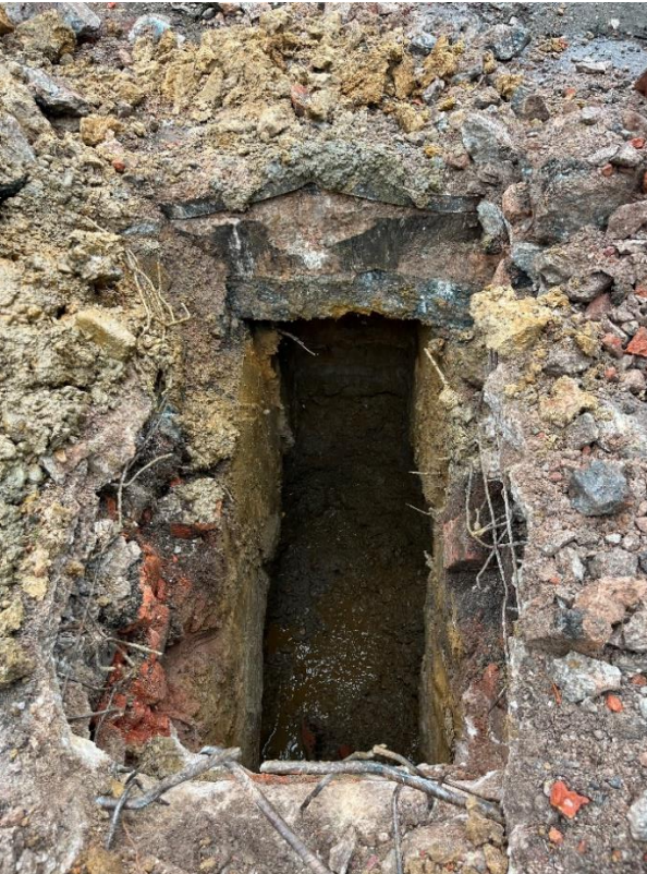
Station Works: 18/07/23 TP04A Complete
