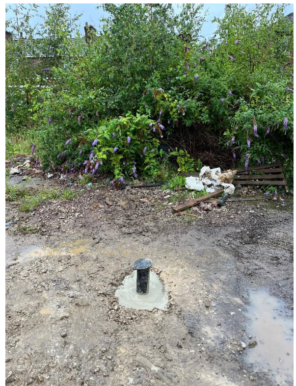
Station Works: 26/07/23 BH04 Install
