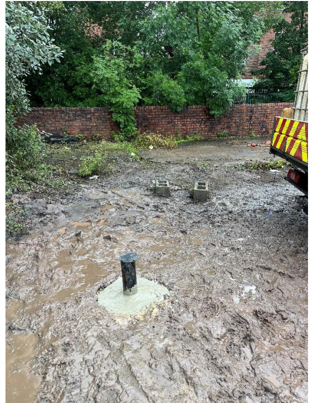
Station Works: 26/07/23 BH02 Install
