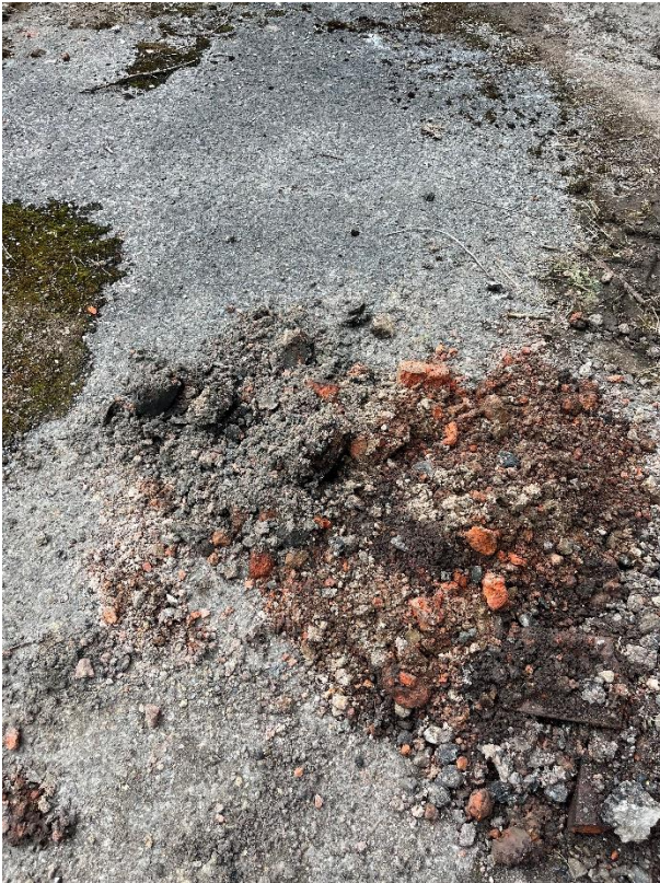
Station Works: 23/07/23 BH02 Made Ground
