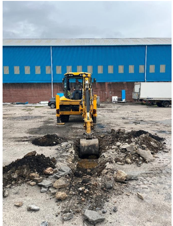
Station Works: 18/07/23 TP01 Made Ground
