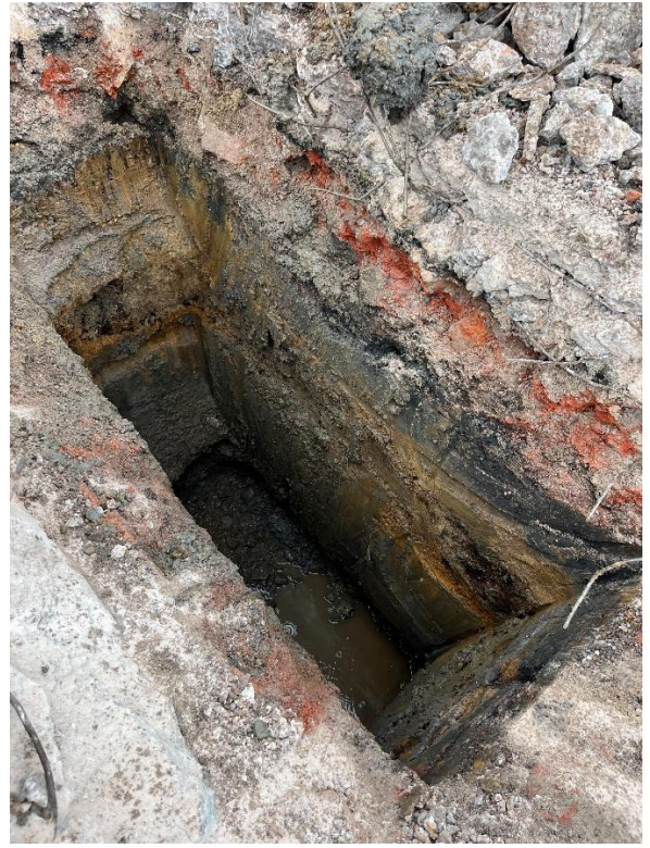
Station Works: 18/07/23 TP03 Side View
