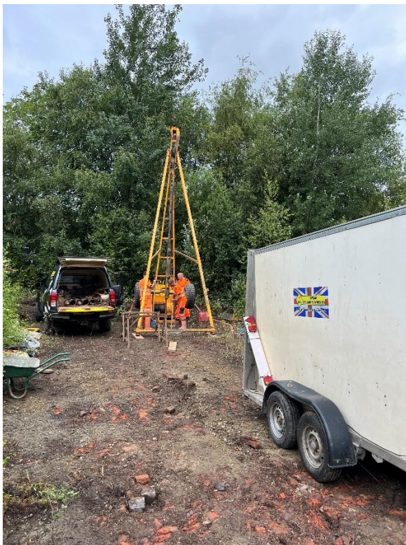
Station Works: 19/07/23 BH01 Location
