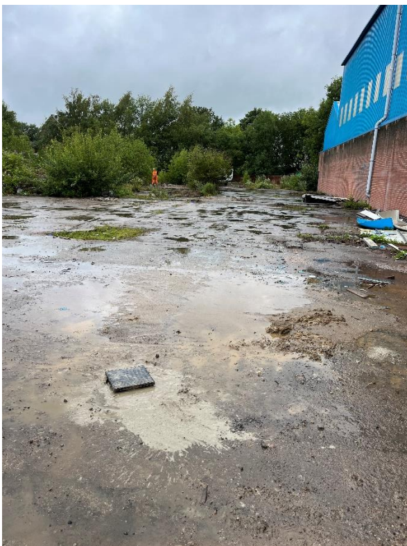
Station Works: 26/07/23 BH03 Install
