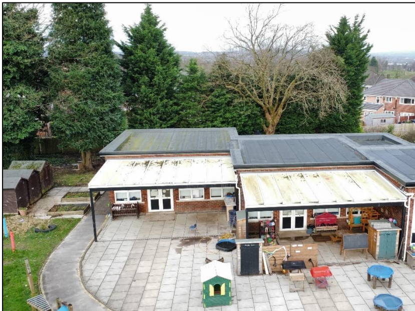
Photograph 1 showing the rear of Building 1
