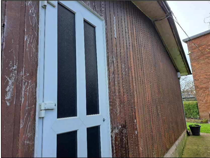
Photograph 4 showing the soffits of Building 2
