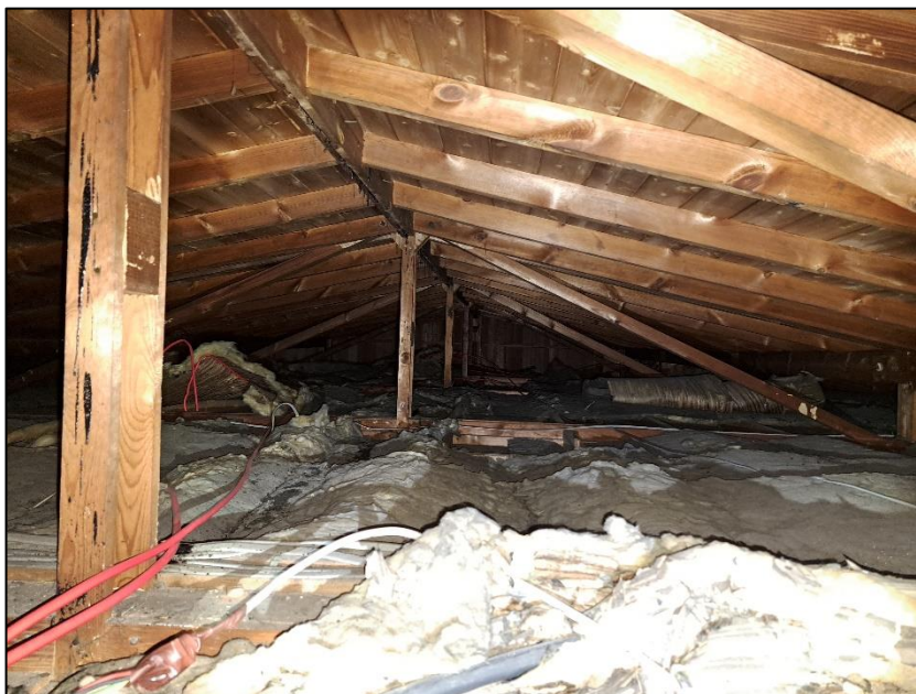
Photograph 6 showing the roof void of Building 2
