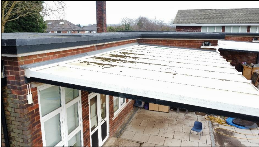
Photograph 2 showing the edge of the roof of Building 1
