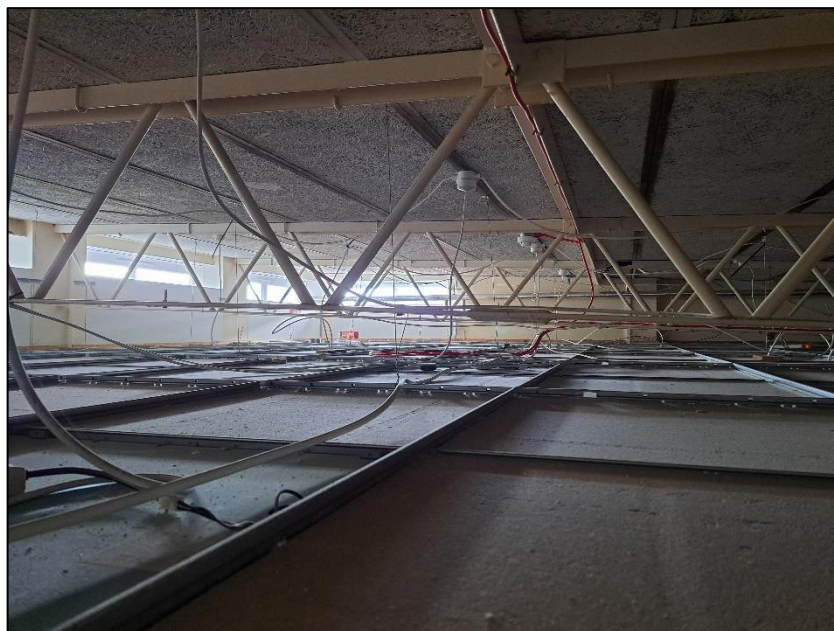
Photograph 5 showing the void above the suspended ceiling
