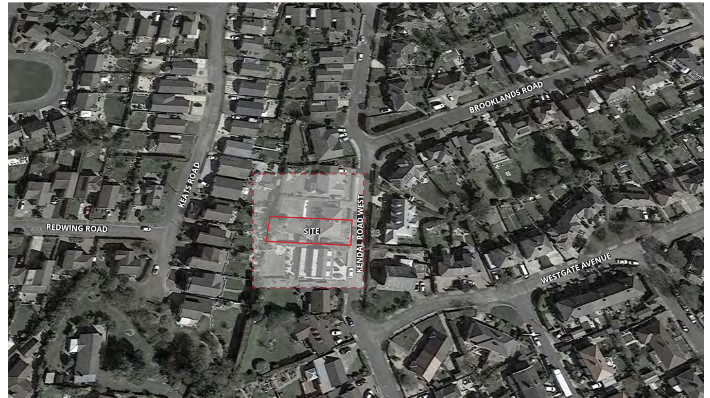
Above: Aerial photograph showing surrounding context
