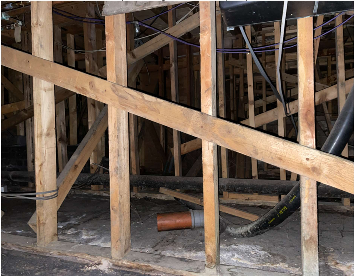
Figure 16- Image of floor void from previous investigation works
