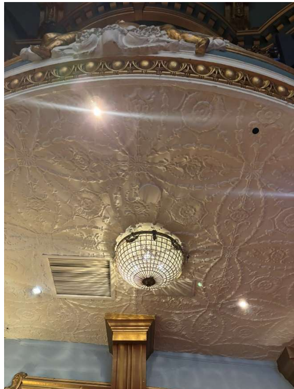
Figure 11 – Decorative plaster work beneath balconies (12.02.2025 Harrison Ince Architects)
