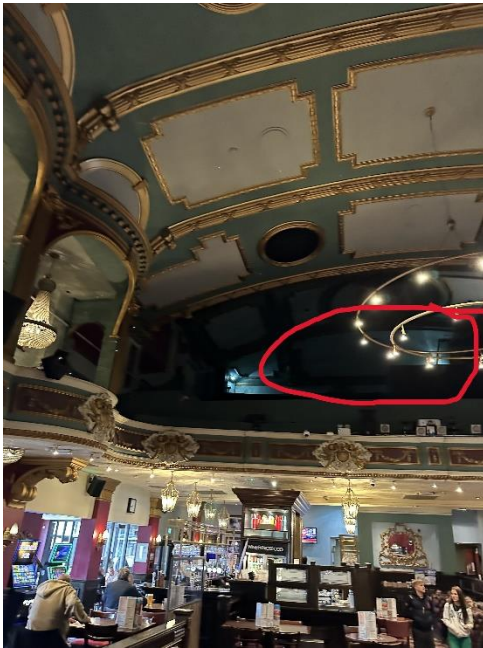
Existing plant in this area removed
