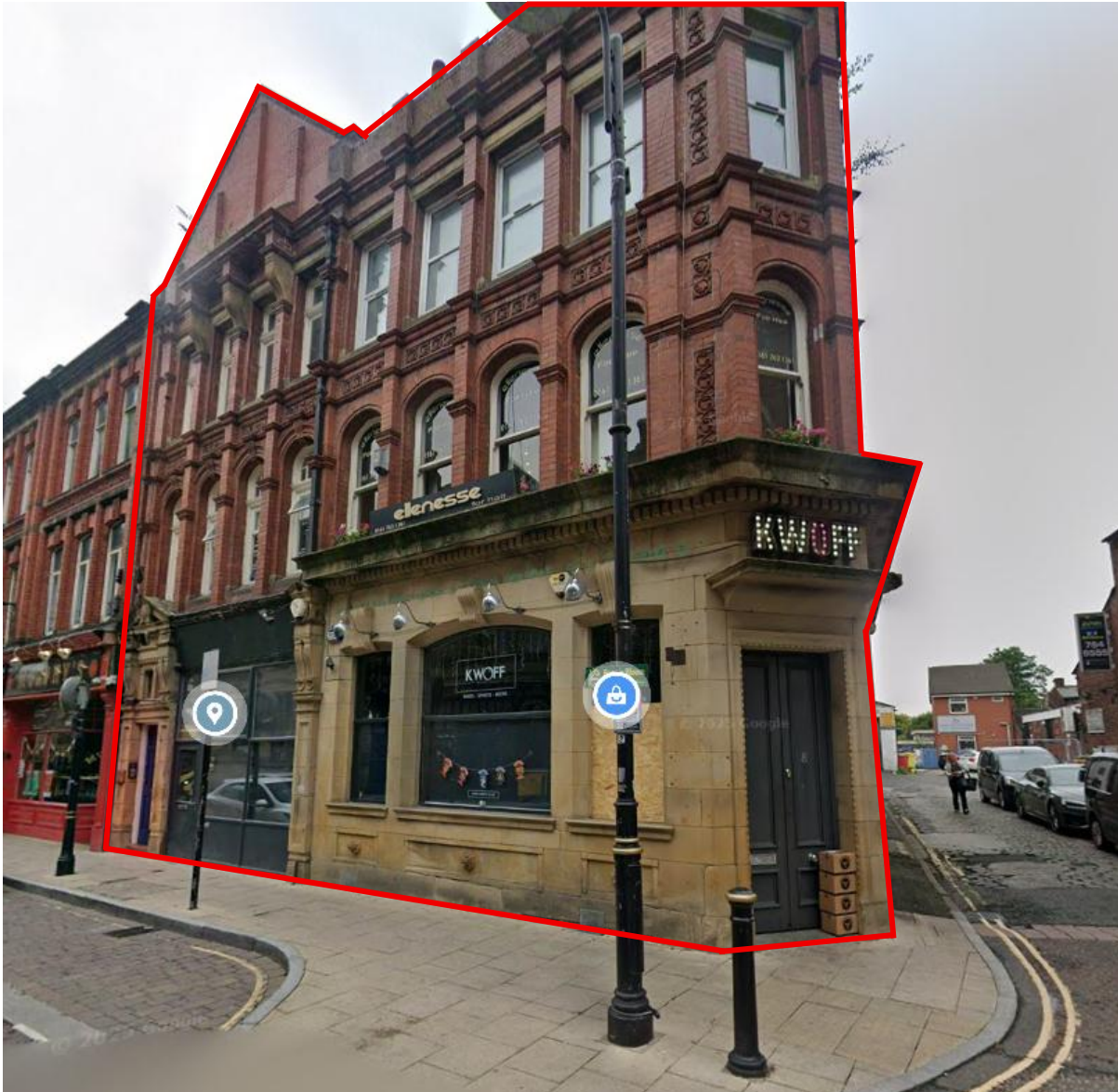
A view of the front of the site, showing any architectural heritage features – that will all be maintained.
