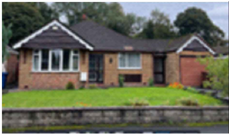
PHOTO WEST ELEVATION
