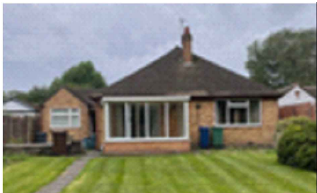
PHOTO EAST ELEVATION
