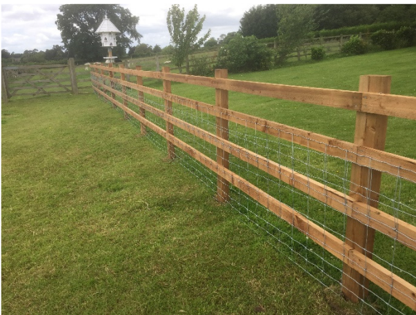
'Post and Rail' Fencing
