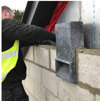
Green and Blue Bat Block/Brick in situ
